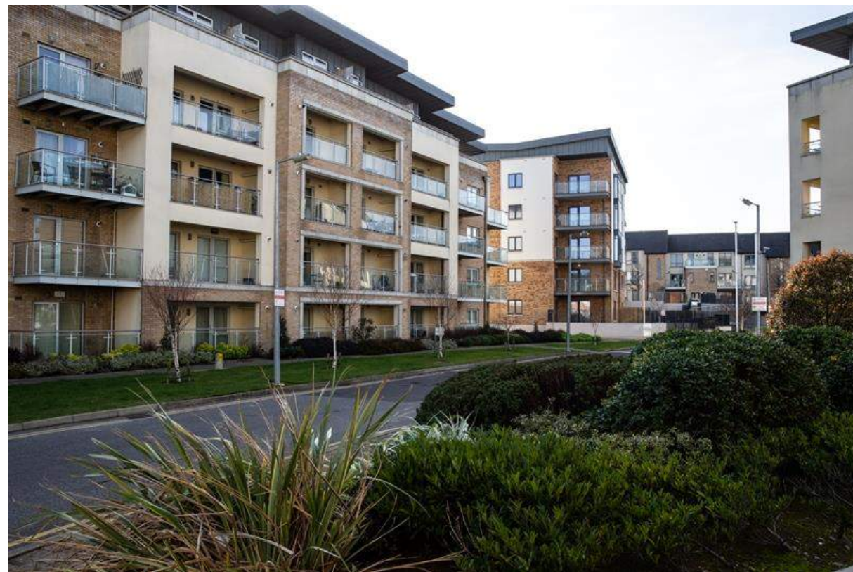
Figure 5.7 – Apartments at Old Glenamuck Road
