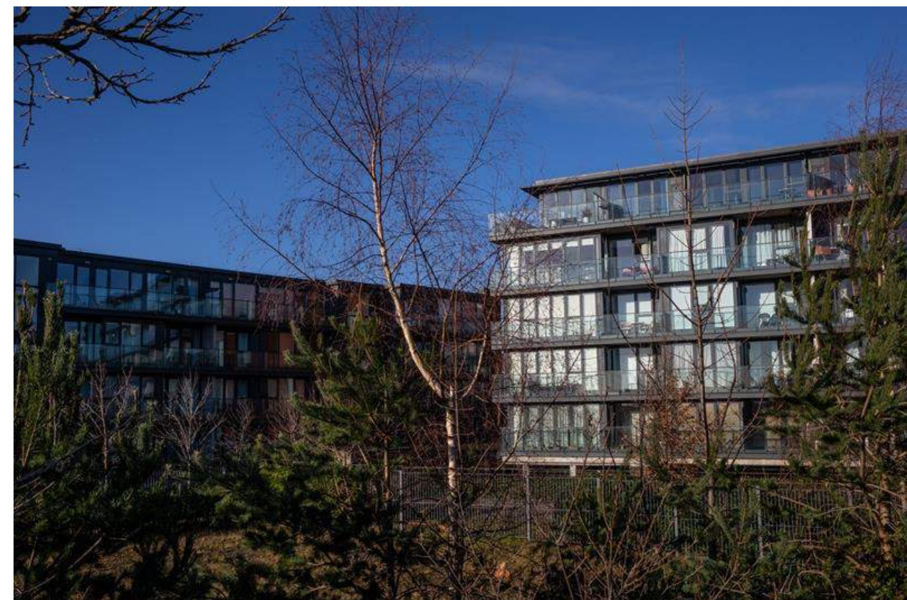
Figure 5.4 – Apartments at Mimosa-Levmoss
