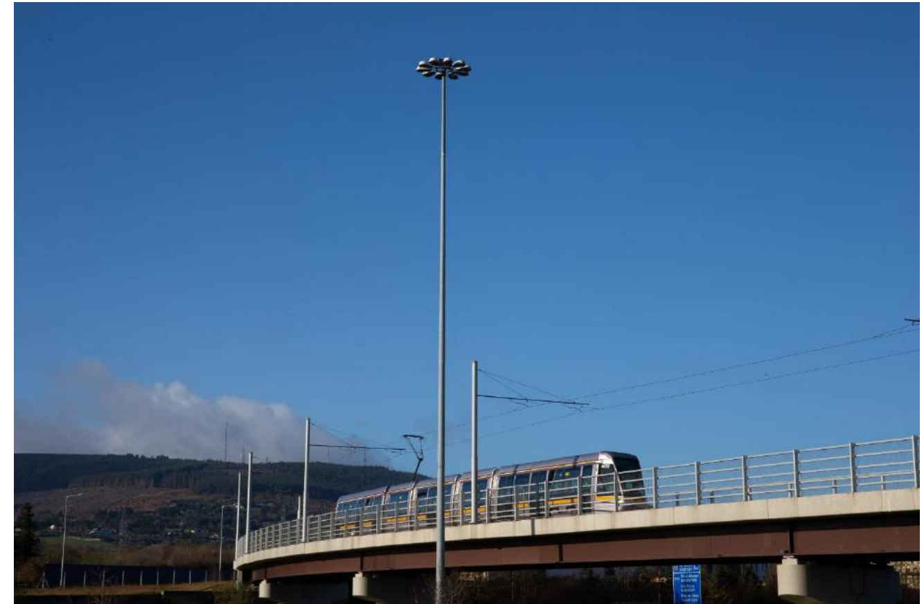
Figure 1.3 – Luas crossing the M50 at Carrickmines
