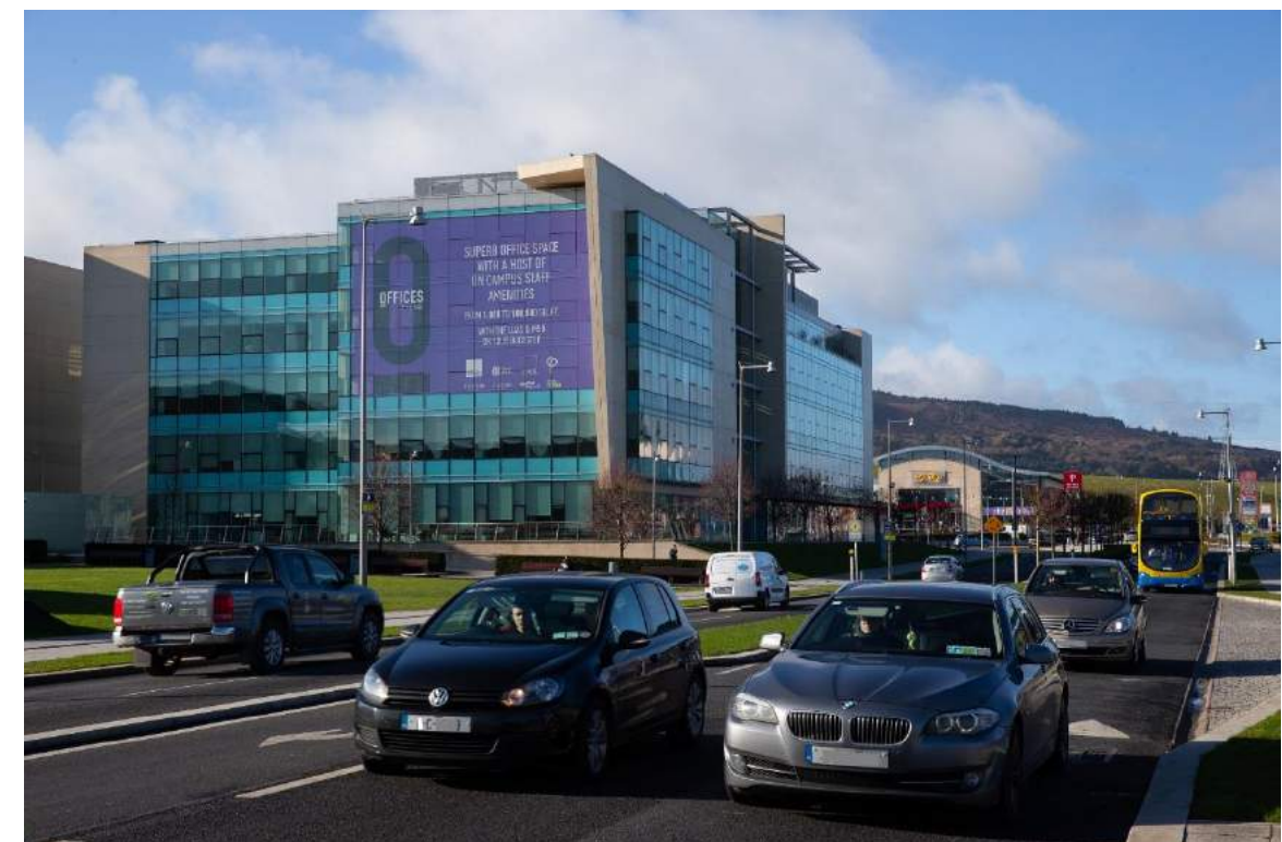
Figure 6.6 - Offices at The Park Carrickmines
