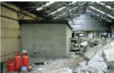
Interior of warehouse, Carlisle Pier.
