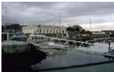
Articulated bridge, Dun Laoghaire Marina.
