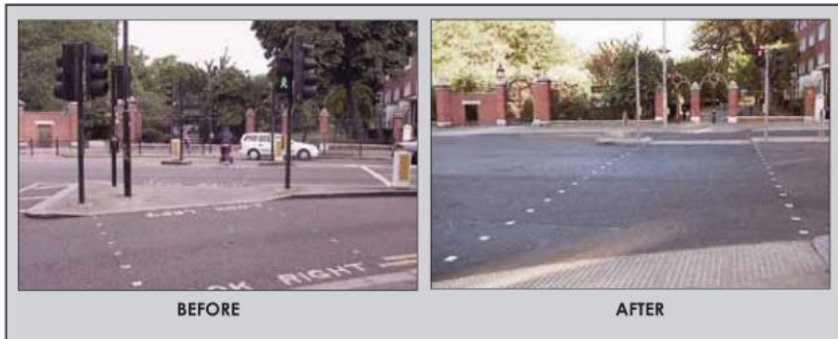
Figure 4.5 Shortened Pedestrian Crossing Distance (DMURS Ref - Fig 4.40)
