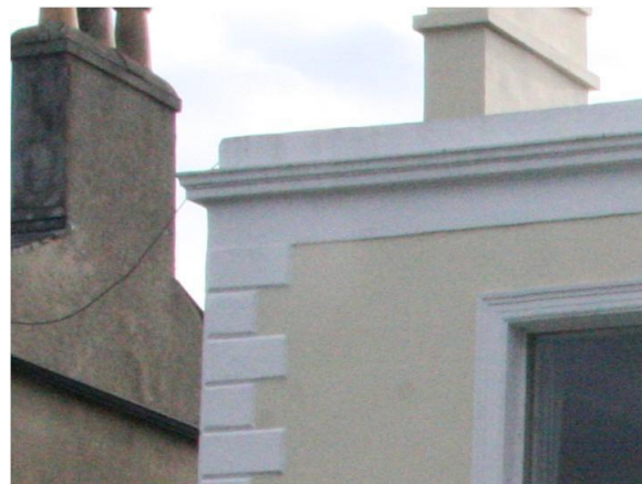
Parapet at Glenmore
