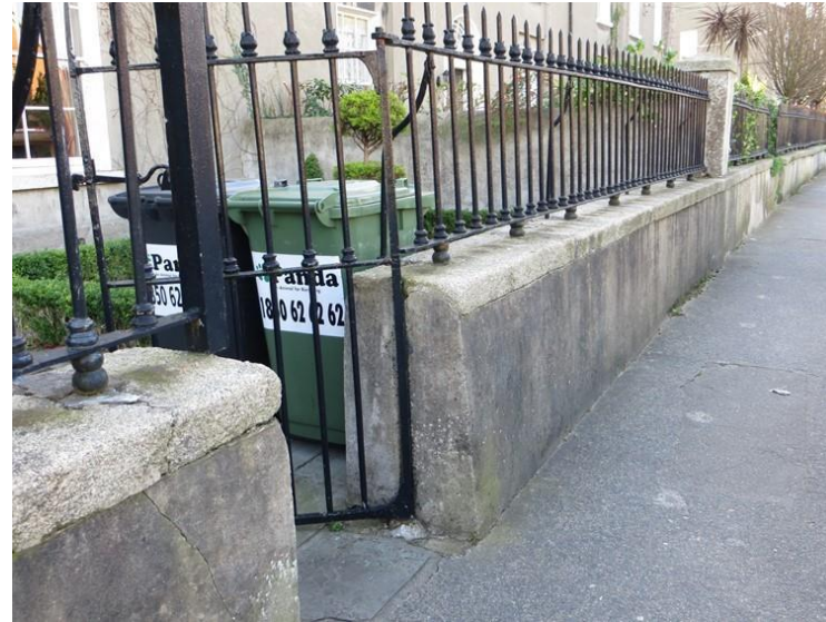
Iron railings on plinth wall, with pedestrian gate
