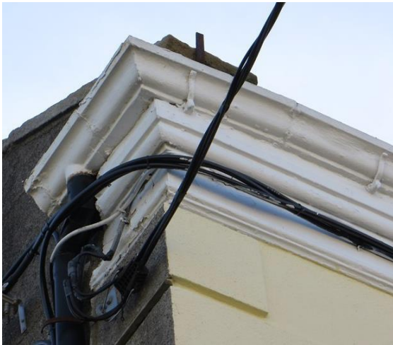
Replacement cast iron gutter
