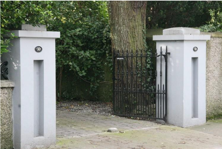
Traditional-style piers and gates at No. 30
