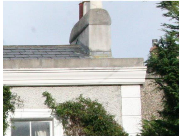
Parapet at Victoria Lodge
