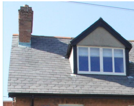
Roof of No. 36
