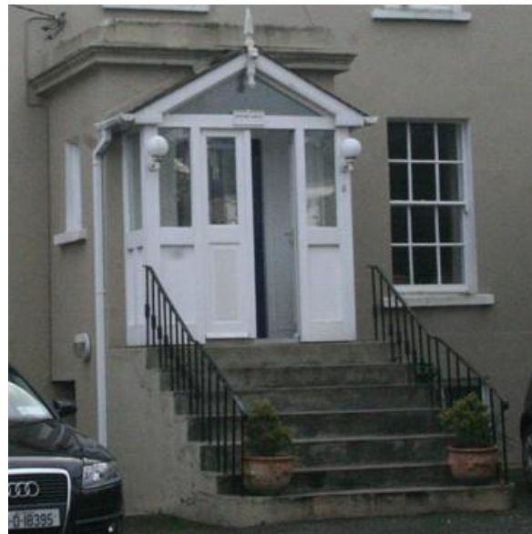
Porch at No. 24
