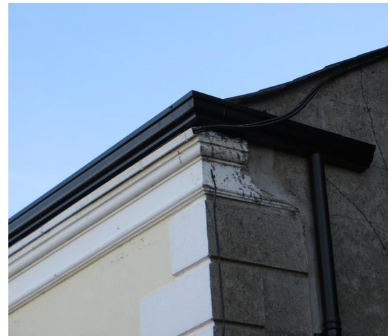
Profiled gutter on No. 2
