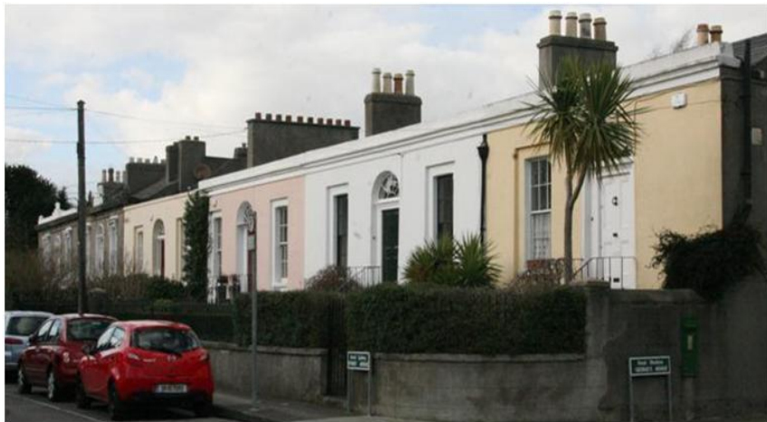
Parapet at Nos. 1, 3 and 5 Sydney Avenue
