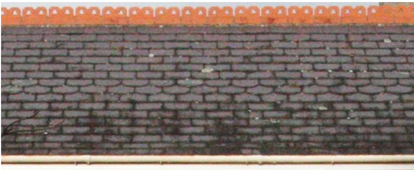
Detail of slates on roof of No. 23 Sydney Avenue
