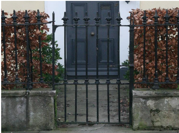
Traditional pedestrian gate at No. 4
