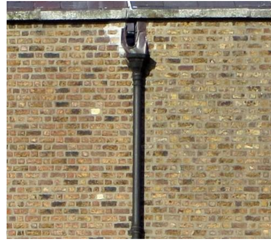
Hopper and downpipe draining from parapet
