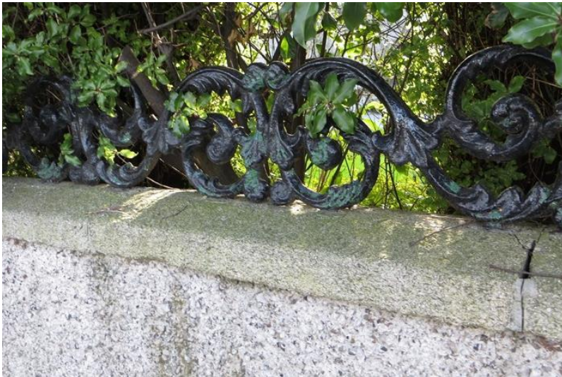
Low cast iron railings on high wall at No. 30
