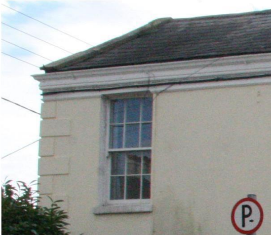
Detail of cornice
