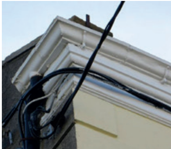
Replacement cast iron gutter
