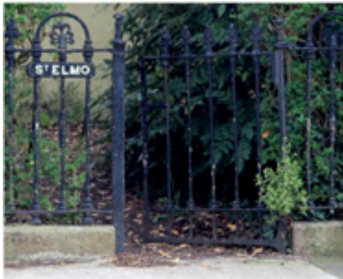
Wrought iron with cast iron details
