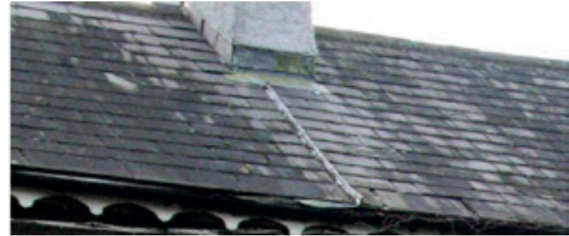
Detail of roof showing wider slates at eaves
