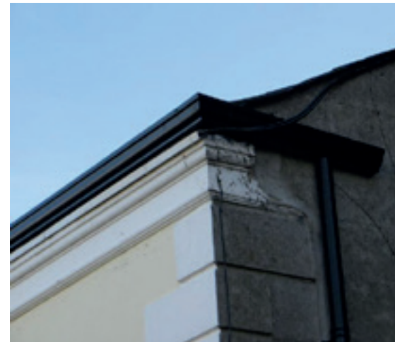
Profiled gutter on No. 2
