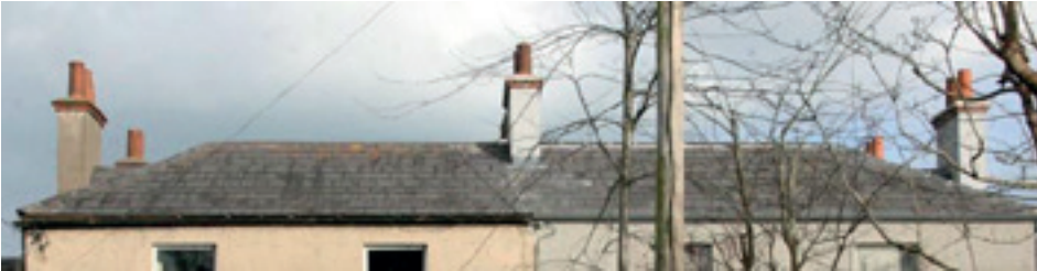
Conical pots and red brick capping
