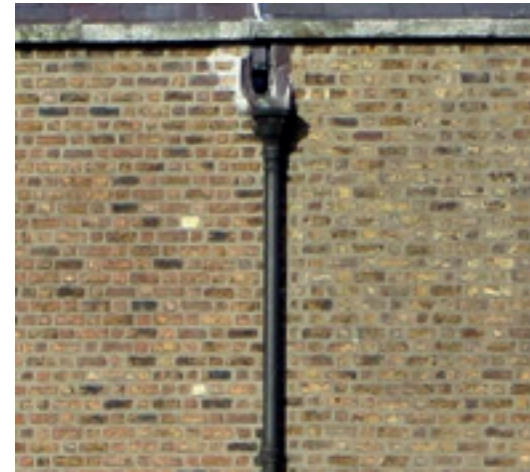
Hopper and downpipe draining from parapet
