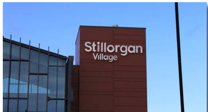
Photo 10: New sign at Stillorgán Shopping Centre
