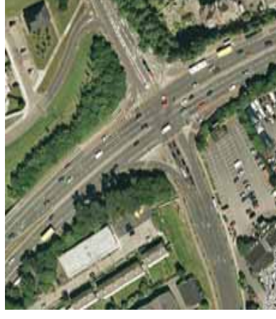
Photo 3.7. Kilmacud Road Lower at Junction with N11
