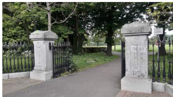
EXISTING VIEW OF GRANITE PIERS
