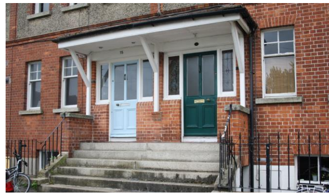
Entrance steps at Nos. 14 and 15
