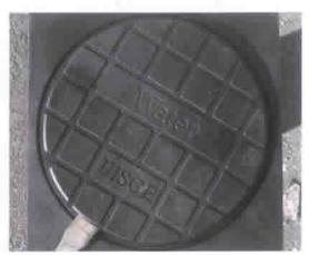
The meter can be opened by prising the lid off. It is important that the meter lid is replaced properly and shut firmly to ensure that the meter box remains water tight.
