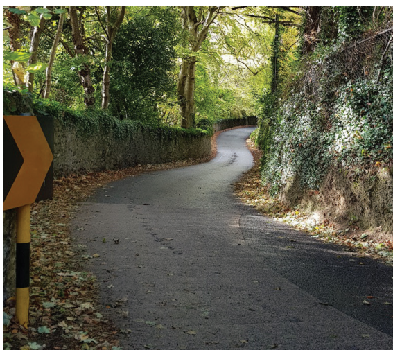
View along Thornhill Road
