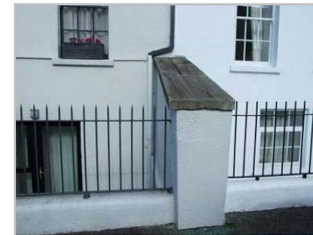
Detail of separating wall and drainage coping between no.4 and no.5
