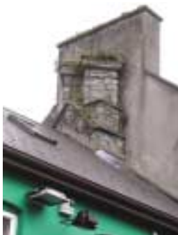
Adjoining buildings that are protected structures may be impacted upon, either directly or visually, although not actually part of the development site. This will be particularly obvious in the case of terraced buildings as in this example which has an important surviving mediaeval chimney stack on a party wall
