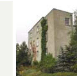
Later extensions of little interest can be carefully demolished without adverse impact on the protected structure as with this later stair tower added to the rear of an eighteenth-century villa
