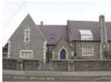
Well-considered extensions can be successfully integrated with a protected structure whether designed in a modern contrasting style (top) or in a matching historicist style (bottom)
