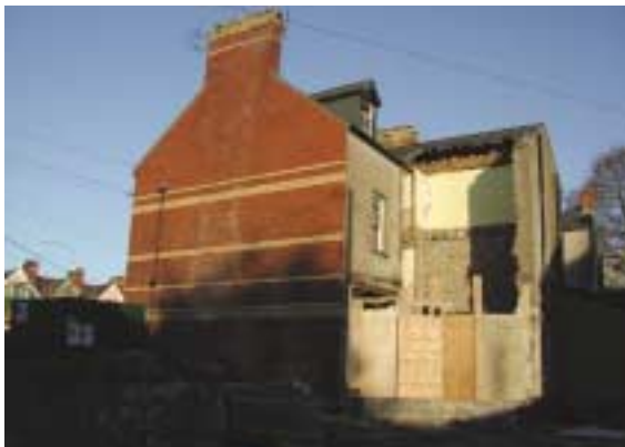
The demolition of a building's return can impact on neighbouring buildings also
