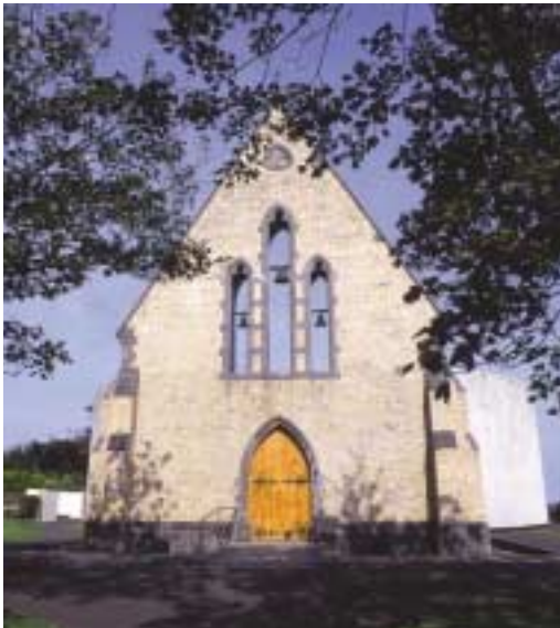
In some cases only part of a structure should be protected as with this church gable wall behind which lies a modern structure
