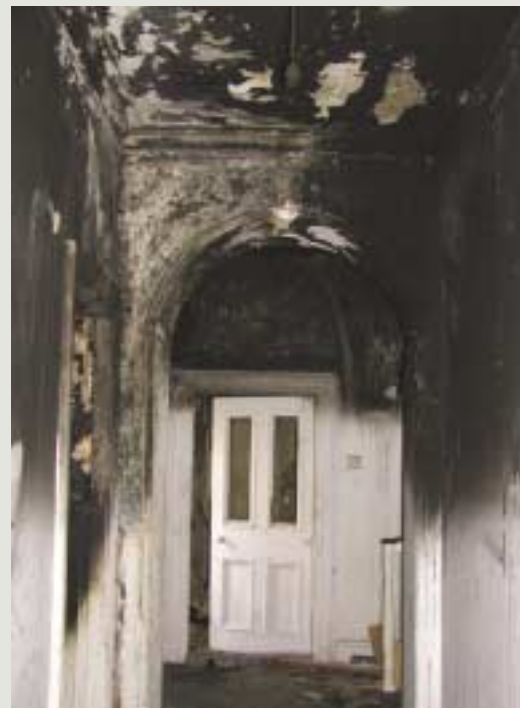
The true extent of damage to important interiors may be disguised by smoke-blackening and blistered paint. Careful spot cleaning of the stained and blistered surfaces and examination of lath and plaster linings will be needed to establish whether or not decorative interior plasterwork or joinery is capable of repair
