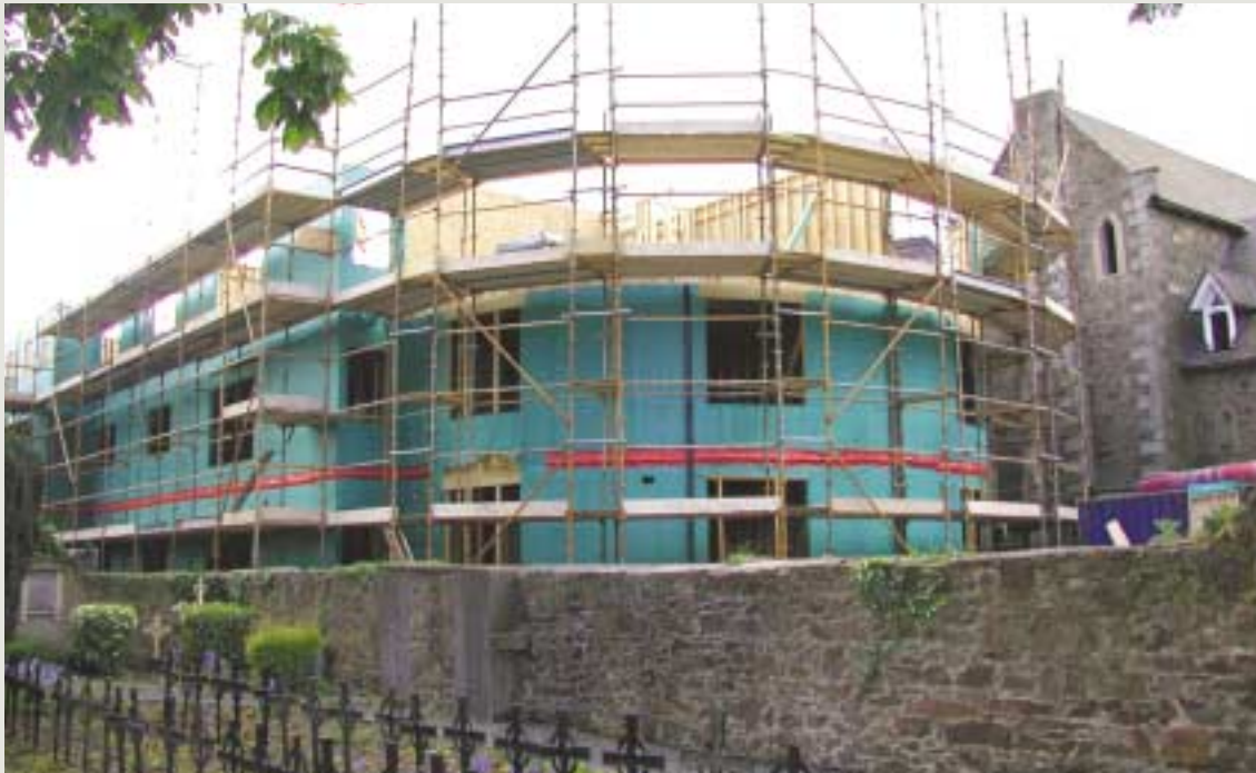
New development in the grounds of this important Gothic revival former convent is under construction between the structure and the nuns' graveyard and has altered their historical relationship
