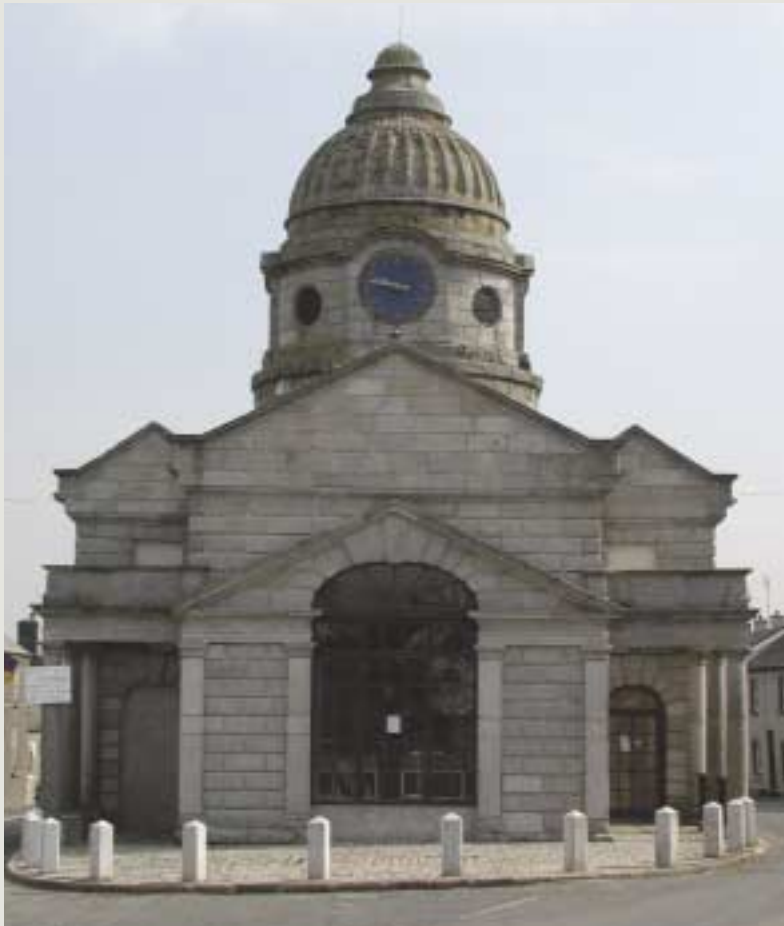
These recent stone bollards, of a plain and robust design, complement, in their solidity and materials, this important courthouse and discourage car-parking against the building and so reduce the potential for damage
