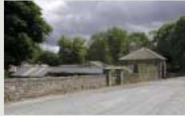
The style and materials of structures used to demarcate the boundaries of a protected structure, its curtilage and attendant grounds can add significantly to its character and that of the surrounding area. This rubble stone wall and fine stone gate piers line the approach to an important complex of stables and farm buildings
