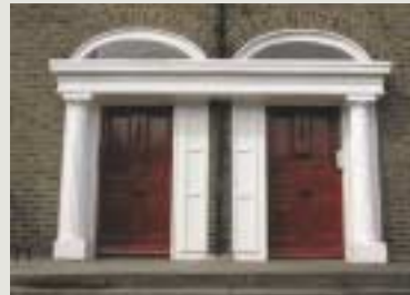
The inaccurately-detailed alteration of doorcases or other features will, in most cases, be to the detriment of the structure and often affect the character of an ACA also
