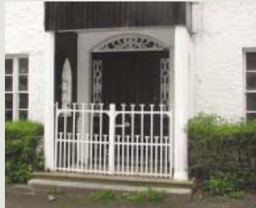
This porch has undergone at least one phase of alteration, although several elements of interest survive, such as point-arched cast-iron windows, strapwork gates and stone steps. Any proposed restoration of a porch such as this should be well detailed, based on good evidence and incorporate surviving features of interest
