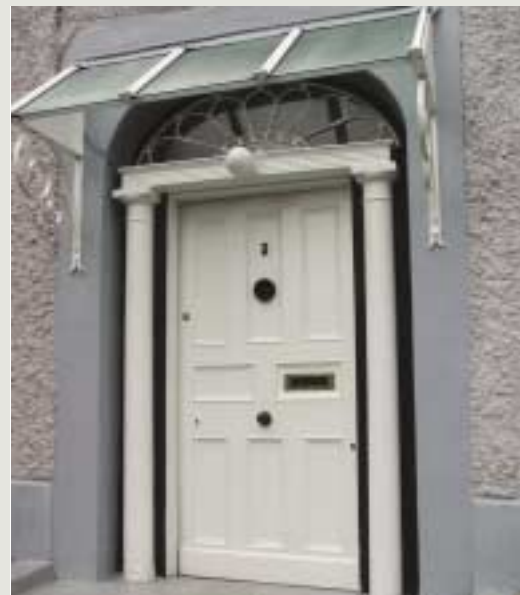
This aluminium canopy is an inappropriate addition to the early nineteenth-century doorcase. Any proposal to remove it should ascertain if the fixings have damaged any cut stonework that might survive beneath the modern render
