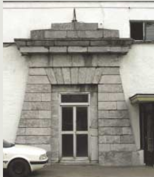
Modern replacement doors of inappropriate design, materials or finishes should not be used. Where such doors now exist, as here, their replacement by an accurately profiled door, informed by research, should be encouraged. Alternatively a high-quality well-designed contemporary solution, which would not adversely affect the character of the historical design, may be acceptable
