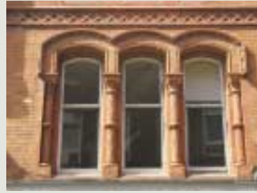
The treatment of structural openings may add considerably to the character of a building; here the elaborate brick and terracotta detailing and the arched window-heads add architectural distinction to the opening
