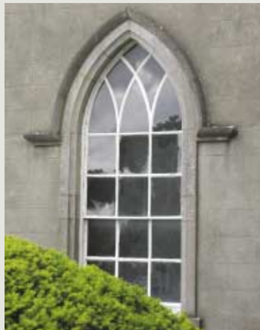
Fully-glazed blind windows such as this example are rare; they may be deliberately designed to ensure symmetrical fenestration (for example, where the plan form did not permit a window), or could represent later blocking of openings. It is commonly thought that openings were blocked to avoid paying window tax, which was in force between 1799 and 1851, however in Ireland there is little evidence to support this theory
