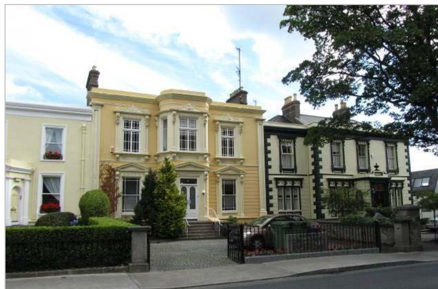
View of No.s 90-91 on Upper George's Street
