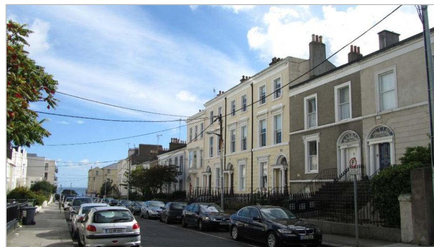
View along east side of Adelaide Street towards the sea
