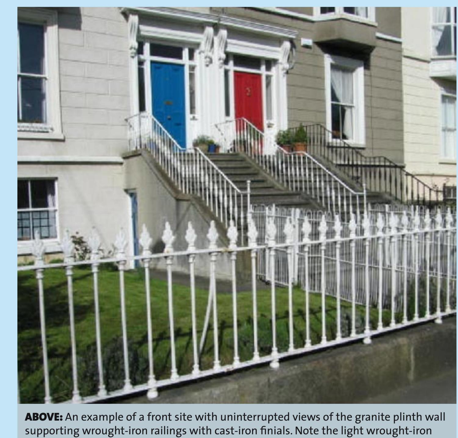
ABOVE: An example of a front site with uninterrupted views of the granite plinth wall supporting wrought-iron railings with cast-iron finials. Note the light wrought-iron fencing which encloses the lawned landscape area from the path to the front door.
