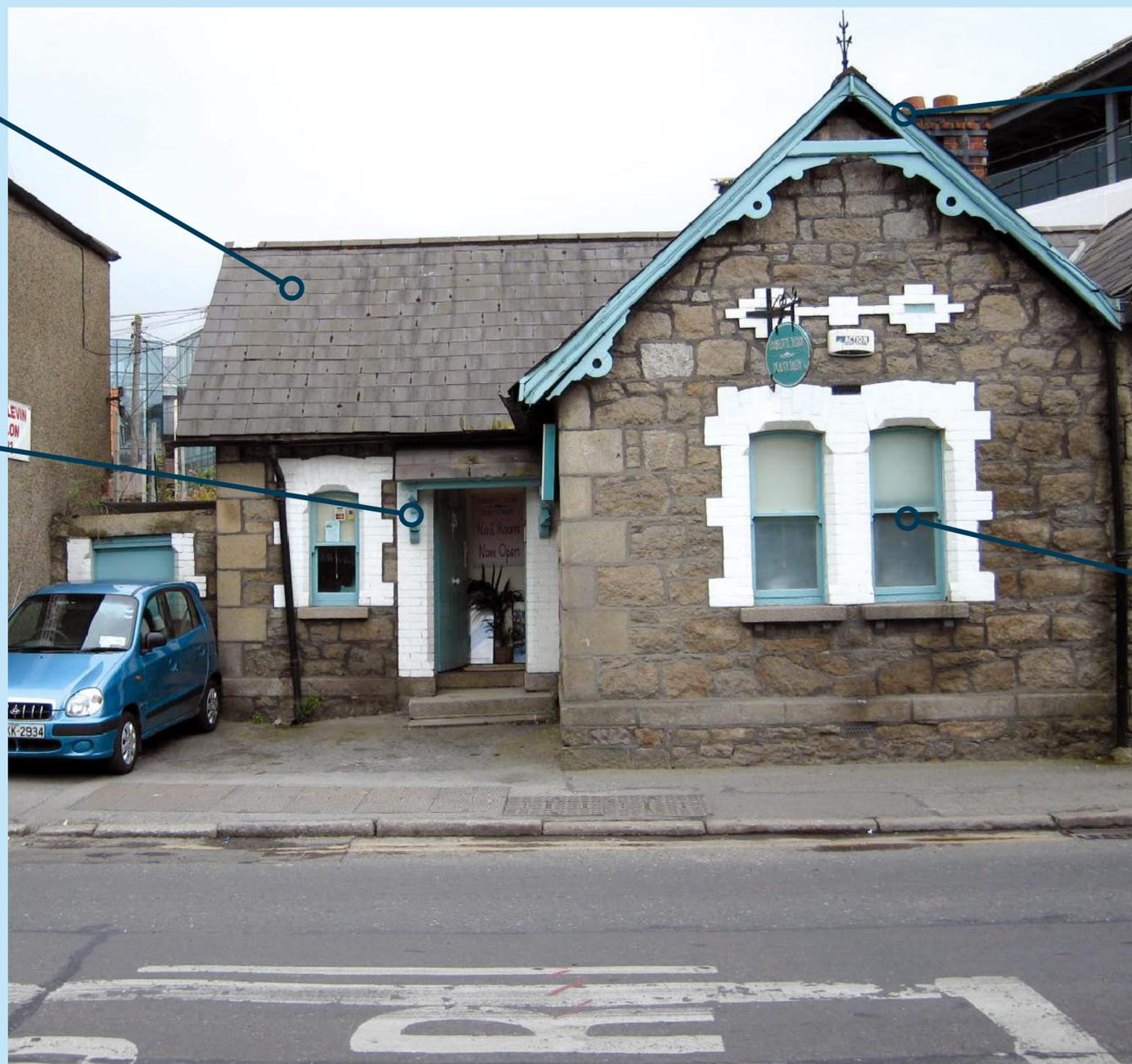
Recovered artificial slate roof. The original roofing material would have been Blue Bangor slates.
