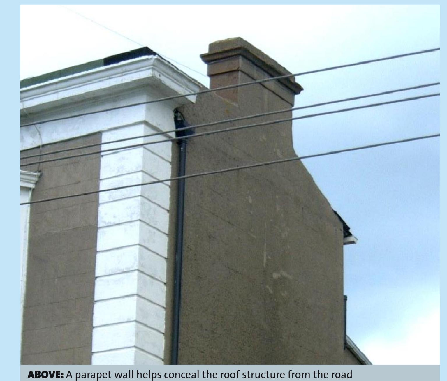
ABOVE: A parapet wall helps conceal the roof structure from the road
