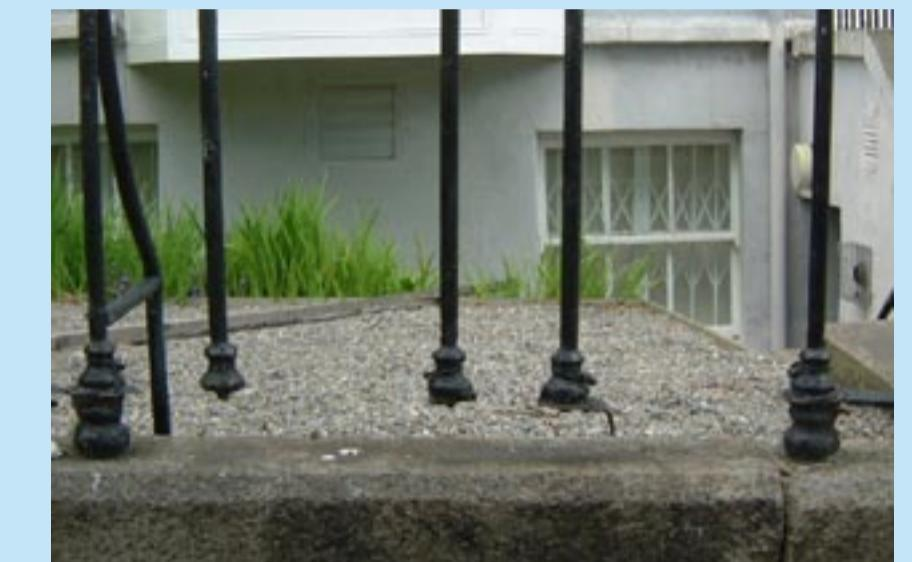
**ABOVE:** The bottom rail of the railing has been broken. It should be replaced to stabilise the upper part of the railing.
