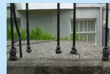
**ABOVE:** The bottom rail of the railing has been broken. It should be replaced to stabilise the upper part of the railing.
