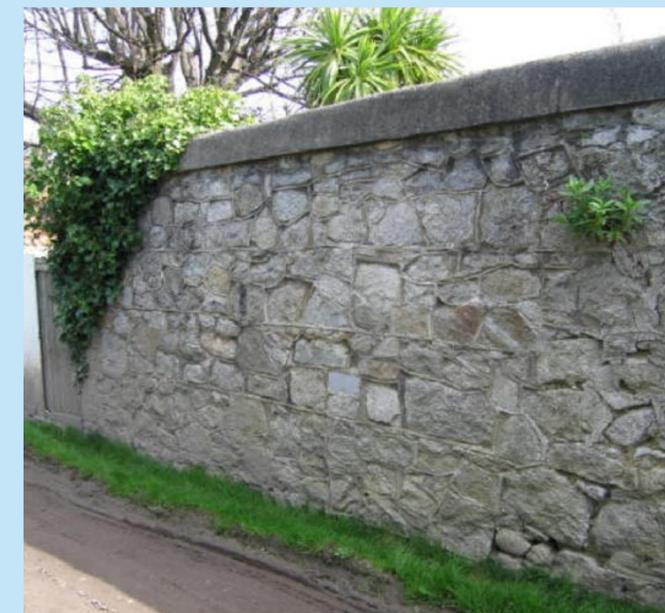
ABOVE: An example of a rubble granite boundary wall with render flanching and rear site pedestrian entrance.
