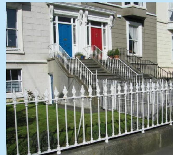
ABOVE: An example of a front site with uninterrupted views of the granite plinth wall supporting wrought-iron railings with cast-iron finials. Note the light wrought-iron fencing which encloses the lawned landscape area from the path to the front door.
