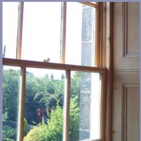
Fig 10. Existing sashes re-glazed with DG units.
