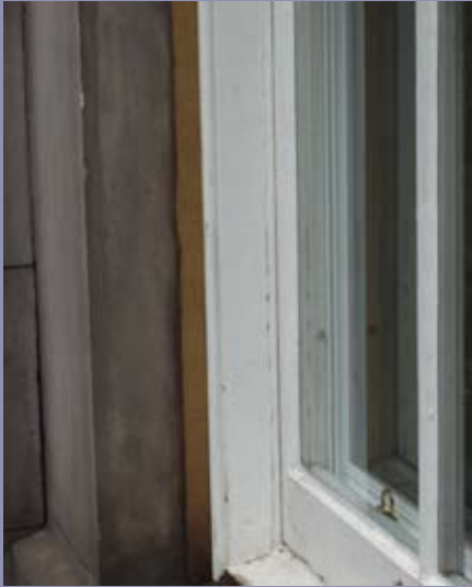
Fig 7. How does it look - Secondary glazing (seen in Fig 6) fitted on a sash window. Changeworks
