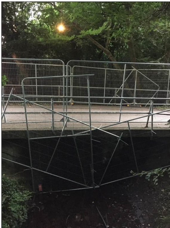
Plate 5: Heras fencing installed on bridges to prevent unauthorised access to event.
