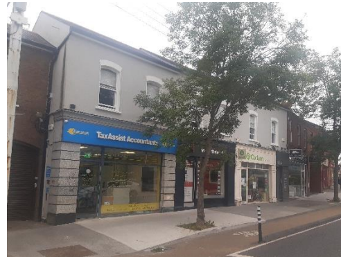
Photo 5.10: Example at Claremont Terrace, northern end of Main Street
