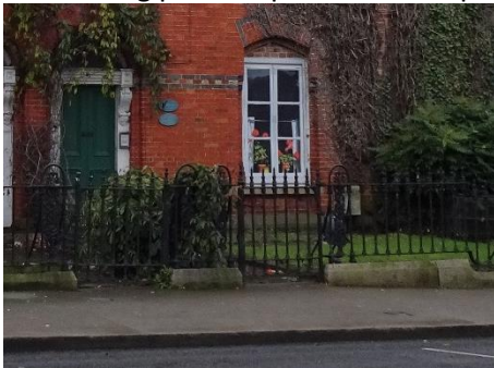
Photo 5.5: Ironwork (gate and fence) to the front of Glenville Terrace, Main Street
