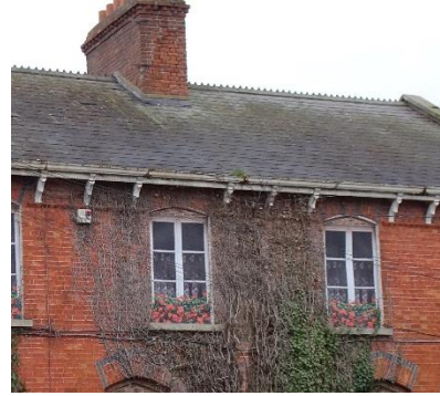
Photo 5.8: Use of slate at Glenville Terrace
