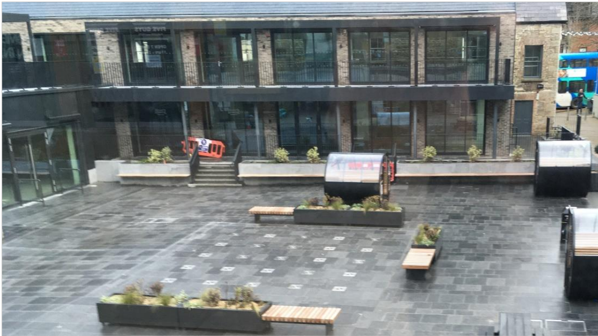
Photo 5.18: Ashgrove Terrace and public space (known as Pembroke Square) following renovations. The 2-storey extension is visible left of frame.
