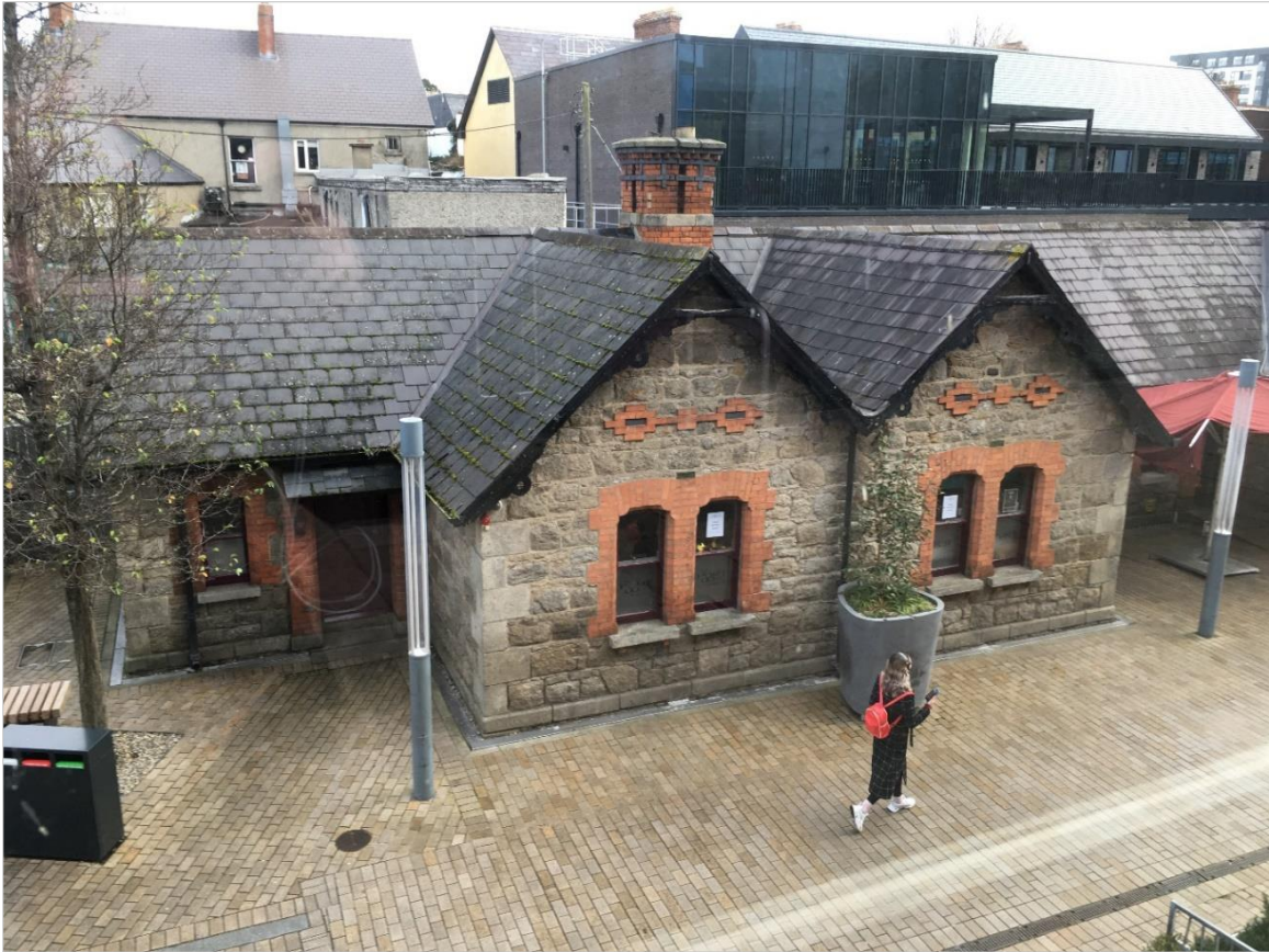
Photo 5.28: Nos 3-4 Pembroke Cottages, part of the 'Pembroke District' (restaurant uses). The units have been combined internally.
