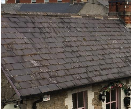
Photo 5.7: Slate in use at 1-2 Pembroke Cottages, Ballinteer Road
