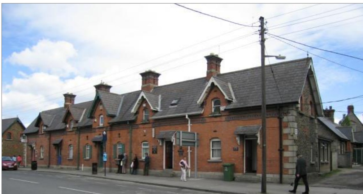
Photo 5.11: Nos. 14 –18 Pembroke Cottages Dundrum.
