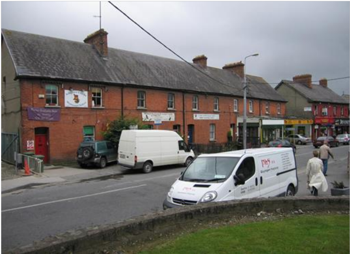
Photo 5.16: Ashgrove Terrace prior to refurbishment
