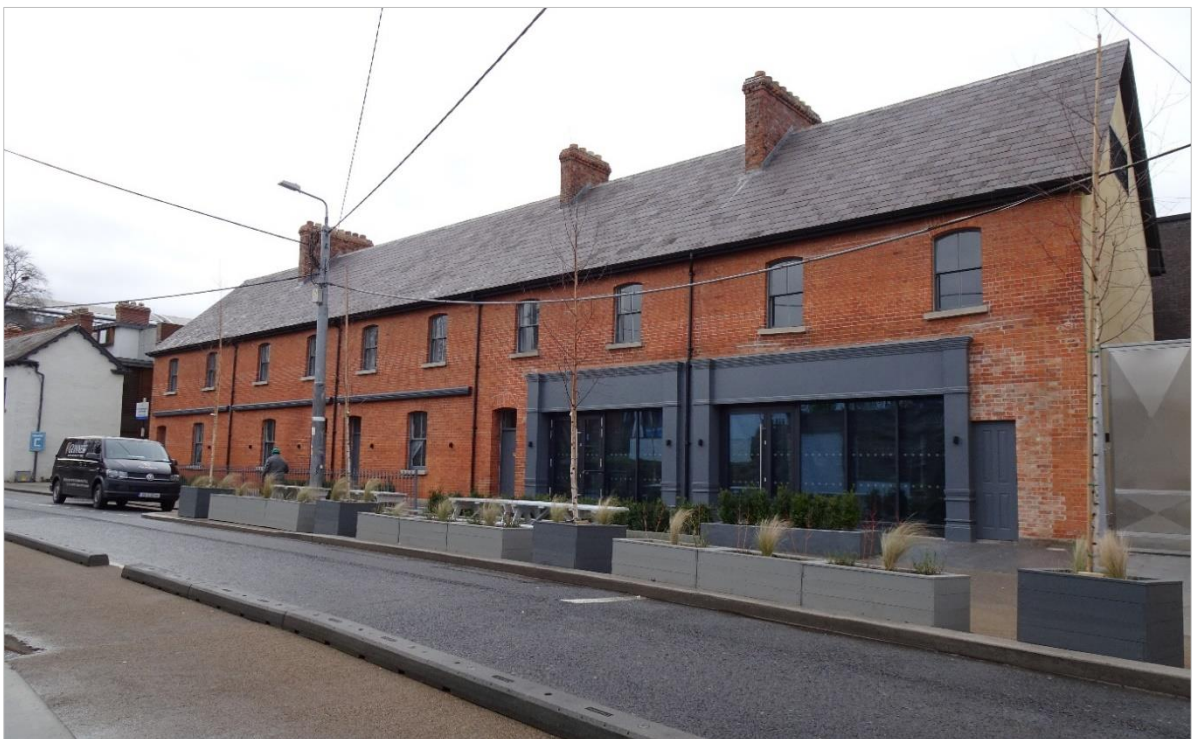
Photo 5.17: Ashgrove Terrace post refurbishment (January 2021)
