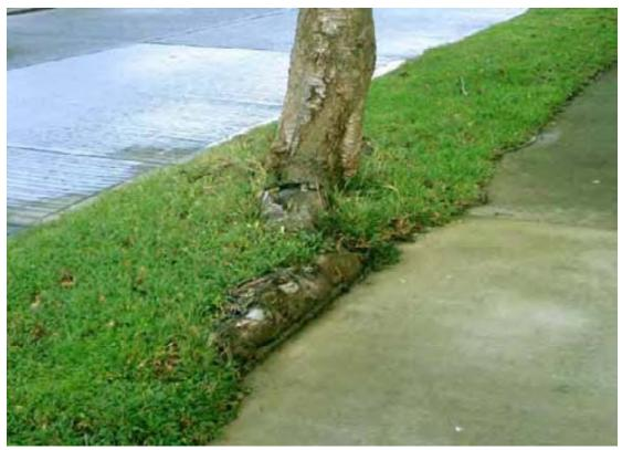
Footpaths are regularly replaced as a result of damage by Cherry tree roots
