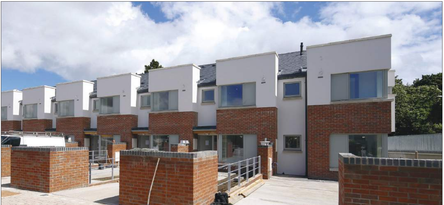
Works under way at Cromlech, Enniskerry Road.
