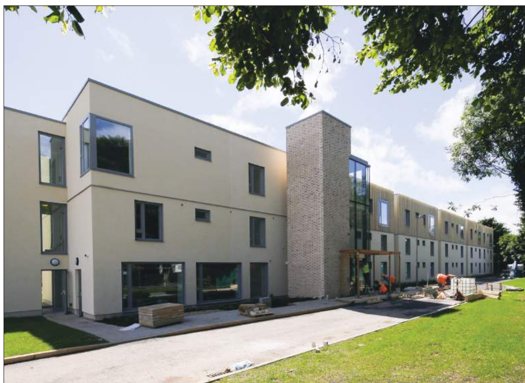
Works nearing completion at Rochestown House Phase 2
