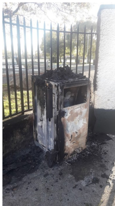
Fig. 3: Bin 365 Loreto Row- after fire
