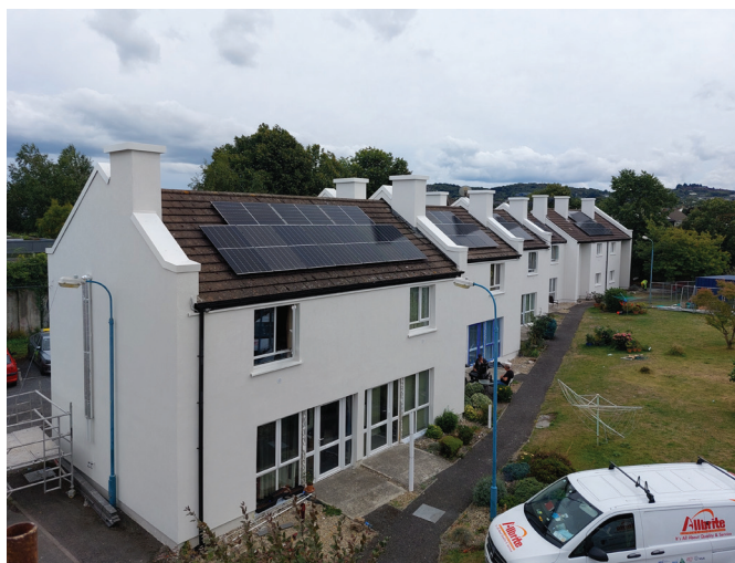
Council housing upgrade works at Beaufort, Glashule
