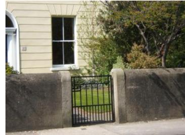
**Fig. 58 Typical pedestrian gate and granite piers**
