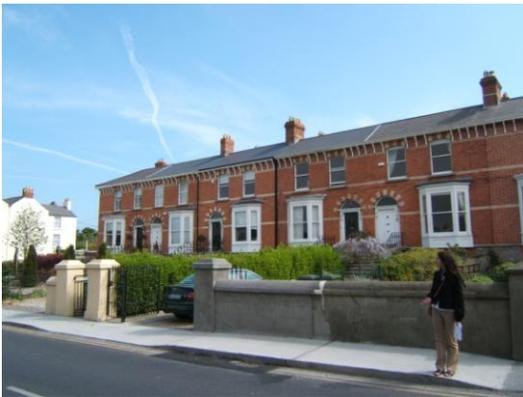
Fig. 17 Mid 19<sup>th</sup> century terrace on Ulverton Road using polychromatic brick, timber bracketed eaves and canted bays.
