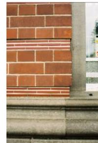
**Fig. 11 Machine cut red brick detail**
