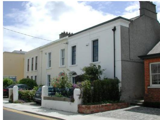
Fig. 18 Rendered terrace on Sorrento Road having moulded architraves and moulded Cornice to the parapet.
