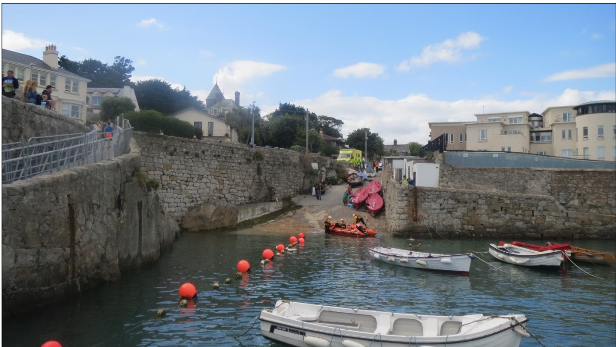
Plate 2: View centred on boat slip from south pier with area of natural rock where works are proposed beneath masonry retaining wall of ramped walkway to left of photograph
