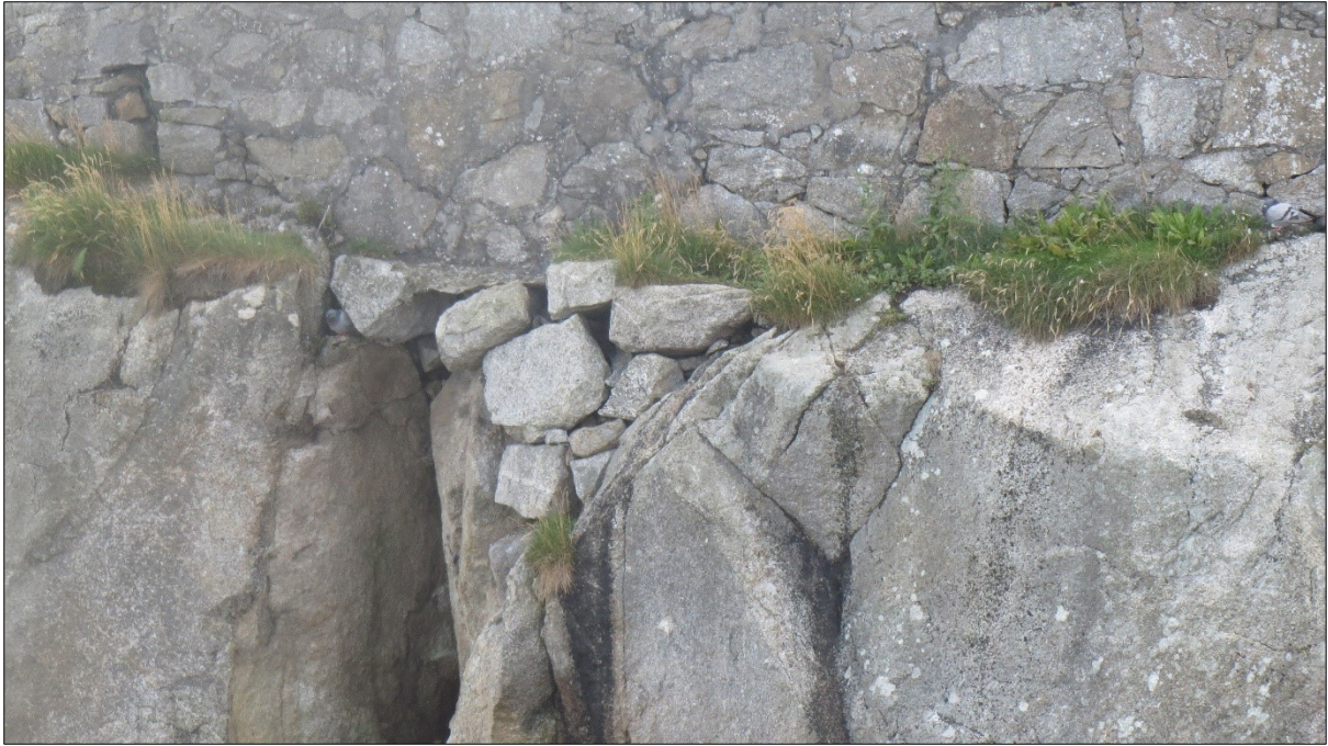
Plate 5: Area of collapsed rock beneath masonry of ramped walkway retaining wall
