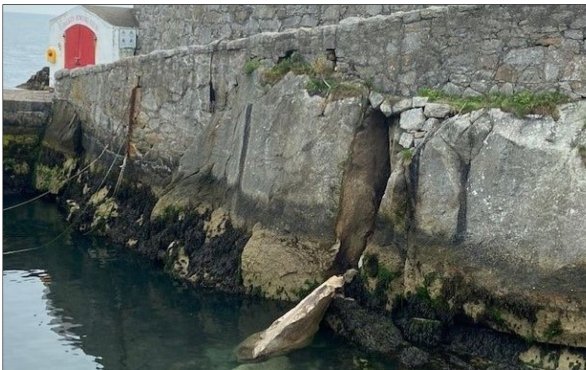
Figure 9: Photograph of collapsed portion of rock forming south wall of Coliemoire Harbour in August 2020 3
