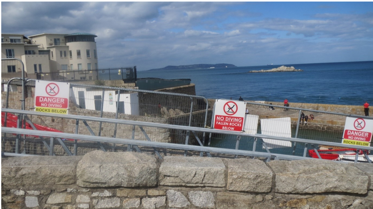
Plate 6: View north over parapet wall to edge of paved area between Coliemore Road and Harbour. Steel hand-rail installed to ramped walkway here in Summer 2021.
