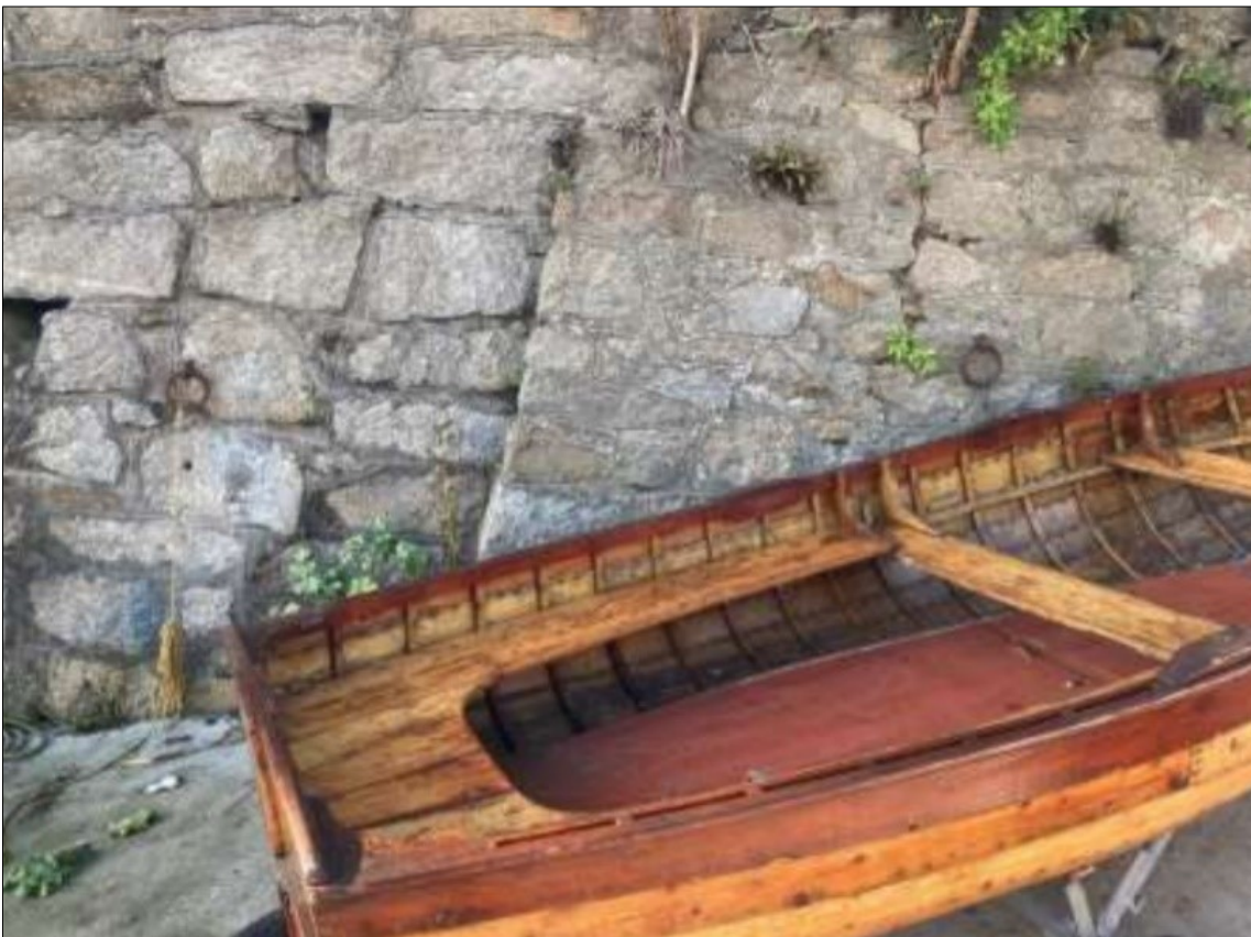
Figure 12: Example of existing metal rings proposed to be fixed to recessed headplates of rock anchors.
