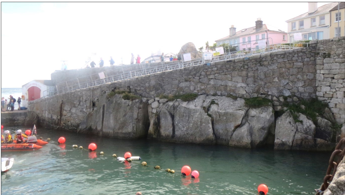
Plate 4: North elevation of rock face to be consolidated as part of proposed works. Rock forms base for masonry retaining wall holding ramped walkway down to former lifeboat house from Coliemore Road. Parapet masonry built with smaller stone and bedded parallel with surface of ramped walkway visible above retaining stonework built directly on natural rock mass.
