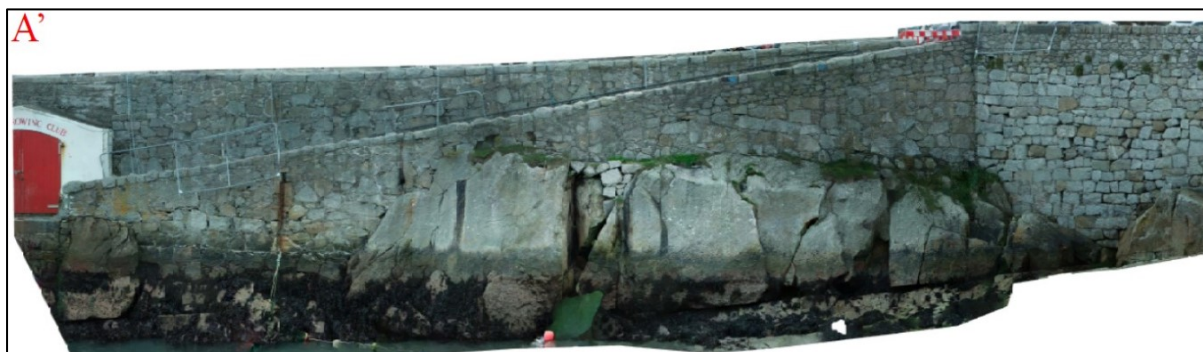
Figure 10: Elevation of existing rock-face supporting ramped walkway between Coliemore Road and south pier of harbour
