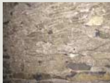
Evidence may survive on a plastered vaulted ceiling or arch of the wicker centring used in forming the vault, seen in the hollows left by the wickerwork which was embedded in the plaster and left there when the centring was removed. In some rare examples, pieces of wickerwork also survive
