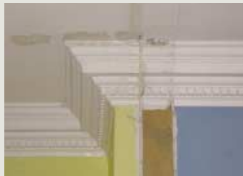
New partitions, where considered acceptable, should avoid disturbing historic fabric. They should be scribed around cornices, dado rails and skirtings to allow removal without damage. However, it is not generally recommended that important spaces within a protected structure be subdivided even if the subdivisions are reversible
