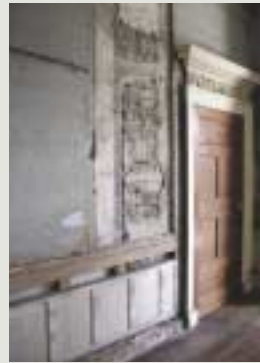
Later finishes or features may cover earlier elements of interest such as this sixteenth-century doorway, partly covered by re-used original panelling and an eighteenth-century doorcase: it may be necessary simply to record the earlier feature while retaining the high-quality later work in place undisturbed
