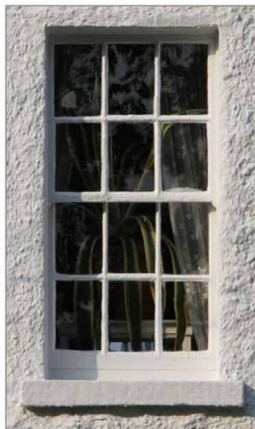
No. 2 also has six-over-six timber sashes, but these do not have the paint accumulation. They may have been stripped and repainted, but the different horns, which are longer and of a slightly later style, suggest that the windows have been replaced.
