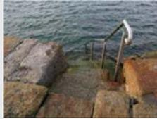
Large unit granite blocks for resurfacing of piers and retaining walls, with historic features retained
