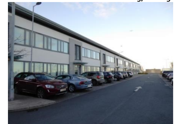
Leopardstown Valley – Office Units to North
