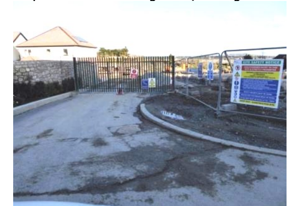
Stepside East – Under Construction at Stepside Park
