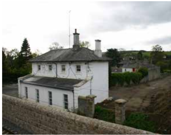
Above: Northern view of building
