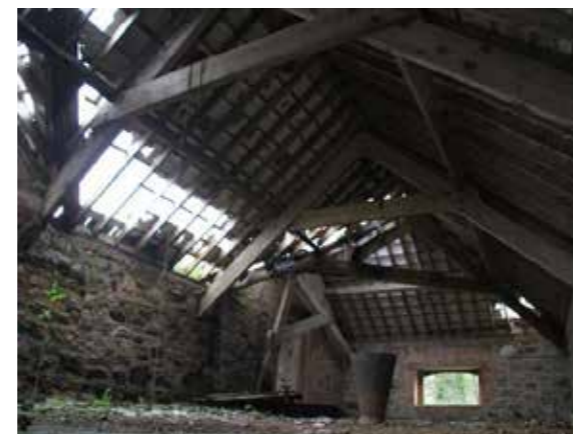
Above: Hay loft with A-truss timber roof
