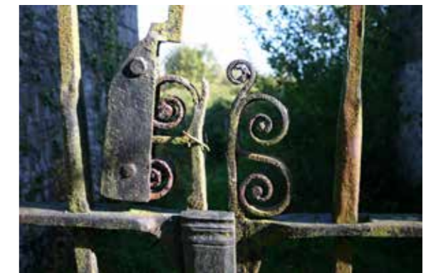
Above: Details of ironwork on gates
