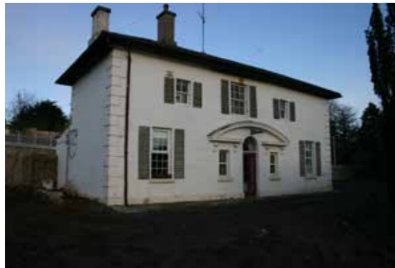
Above: Southern elevation of former station
