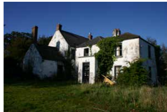
Above: Southern elevation of Lehaunstown Park
