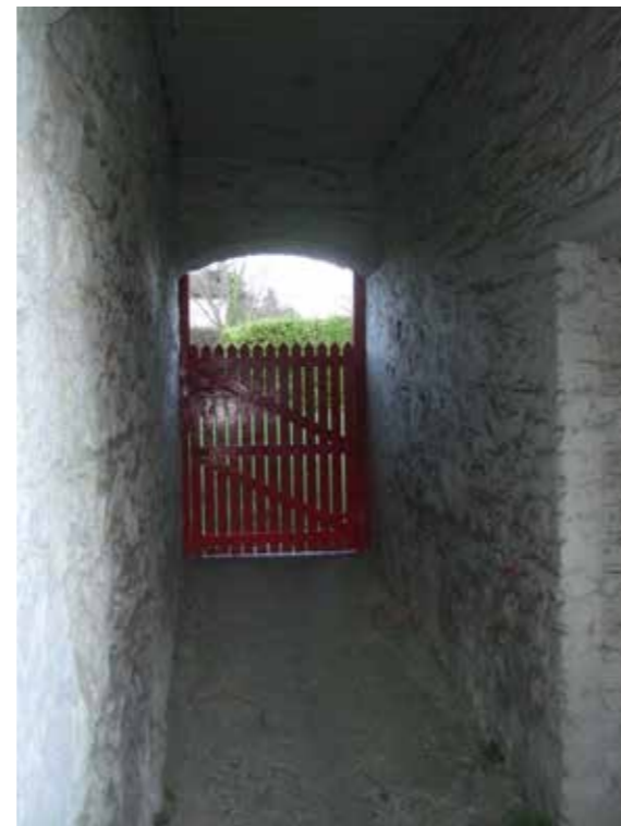
Above: Entrance from stable yard to gardens
