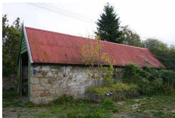
Above: Granite structure on northern side of stable yard
