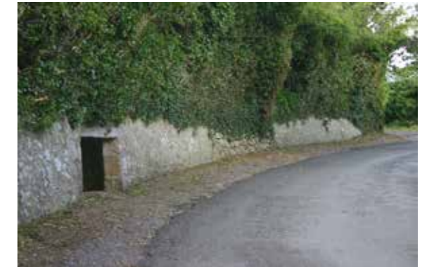
Above: Possible well, Lehaunstown Lane
