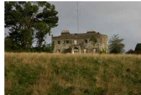
Above: View of front of Glendruid
