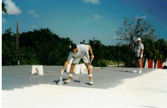
Figure 150. Roof whitening. Source: www.fsec.ucf.edu
