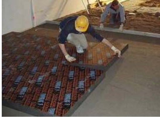
Figure 130. Installation of internal insulation. Source: www.foamglas.es .
