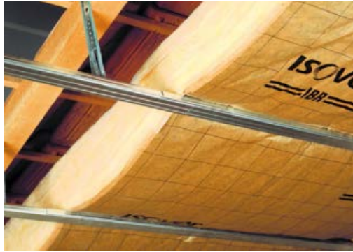
Figure 128. Installation of internal insulation. Source:www.isover.es .
