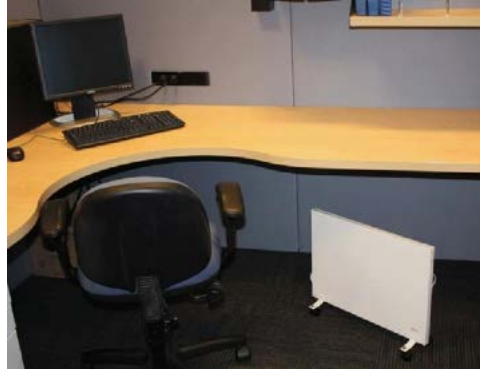
Figure 32. Personal heater in an office. Source: www.facilities.unsw.edu.au .
