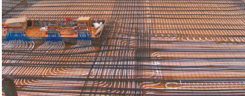
Figure 200. Building a slab with TABs system. Source: www.fenercom.es .
