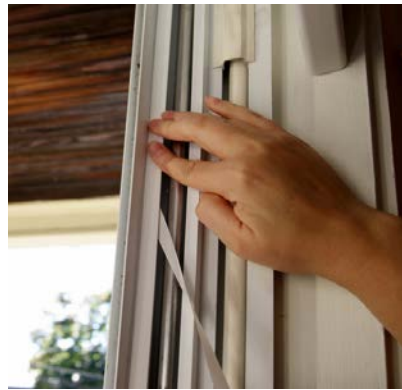
Figure 2. Adding weather stripping at leaky doors and windows. Source: www.imaginecodesignblog.com .
