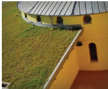
Figure 146. CIRCE's building green roof. Source: Elaborated by CIRCE.
