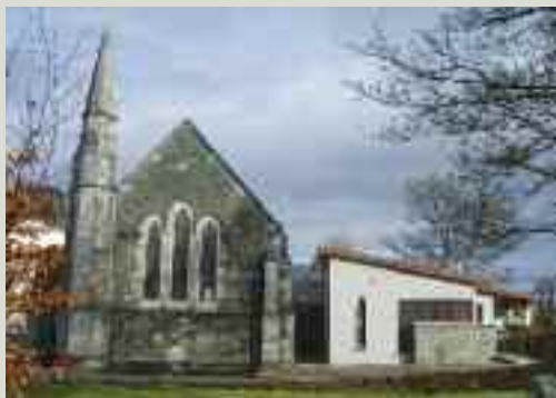
The Methodist Church, Killarney, County Kerry was extended to provide pastoral facilities. The extension was designed in a contemporary style that complements the original historic fabric (Image courtesy of Mott MacDonald Ireland Ltd)
