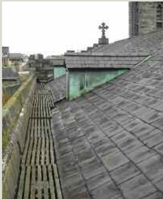
The failed copper guttering and parapet flashings on this church (left) were replaced with new copper guttering and flashing and the stone cleared of growth (right). The snow, or access, boards were not replaced as these can constitute a significant trip or fall hazard at roof level, particularly when they are in poor condition
