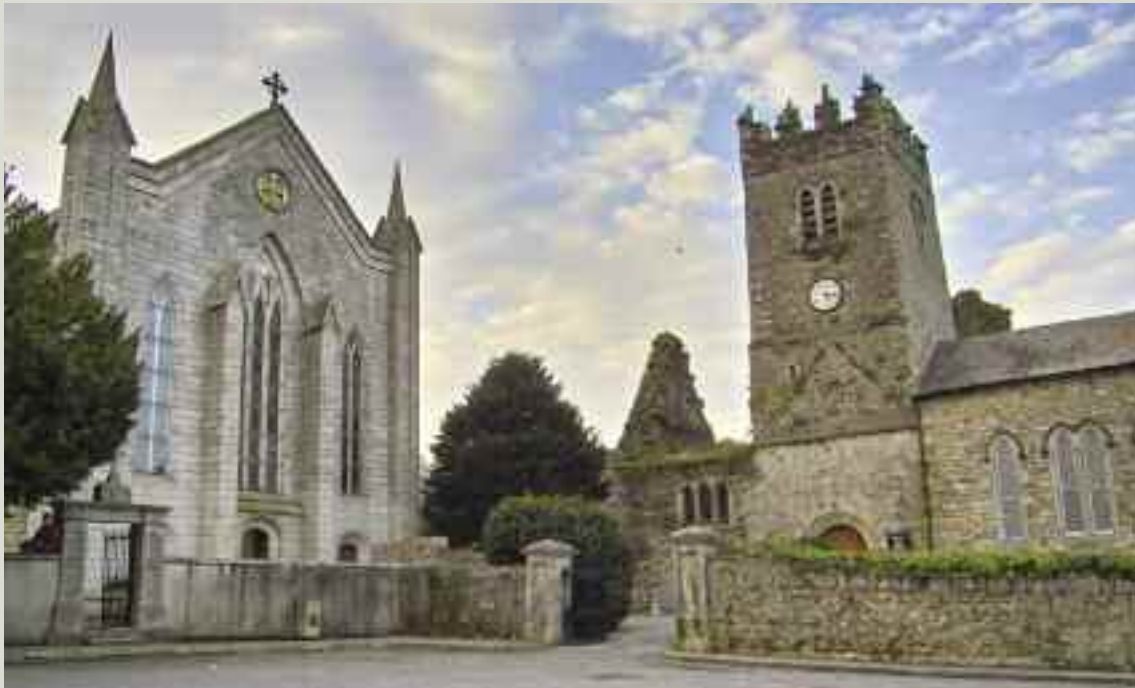
In Inistioge, County Kilkenny, two churches occupy the site of the early thirteenth-century Augustinian priory of Saints Mary and Columba. The priory, Saint Mary's Church of Ireland church (largely altered by the Board of First Fruits in 1824), and Saint Columcille's Roman Catholic church, 1836 (also known as Saint Michael's and as the Church of the Assumption) together form an ecclesiastical quarter within the village
