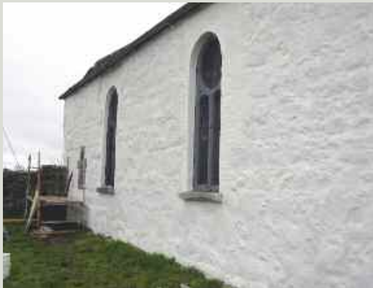
The rubble walls on this medieval parish church were stripped of roughcast cement render and re-rendered using a soft lime mortar. This helped the interior of the building to dry out, assisting to preserve the significant Romanesque stone carving
