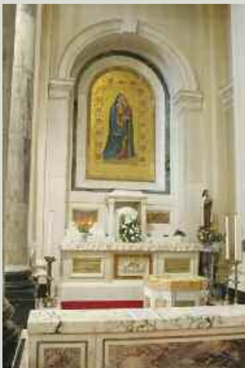
This richly decorated Neoclassical baptistry is separated from the body of the church by Connemara marble columns, which have polished black limestone plinths. The Carrara marble-clad niche houses an Italian gold-leaf mosaic panel
