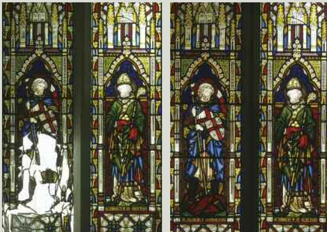
The damage to this window (left) was extensive. Repair (right) consisted of lamination of fractured panes, introduction of carefully chosen and painted intrusions, and re-leading the panels using all surviving pieces
