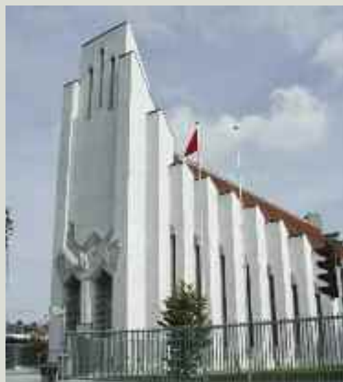
The Church of Christ the King was designed by American architect F Barry Byrne who had trained with Frank Lloyd Wright in Chicago. Constructed in reinforced concrete using strong geometric forms, the church was built to cater for the growing Catholic population in the expanding suburbs of Cork City
