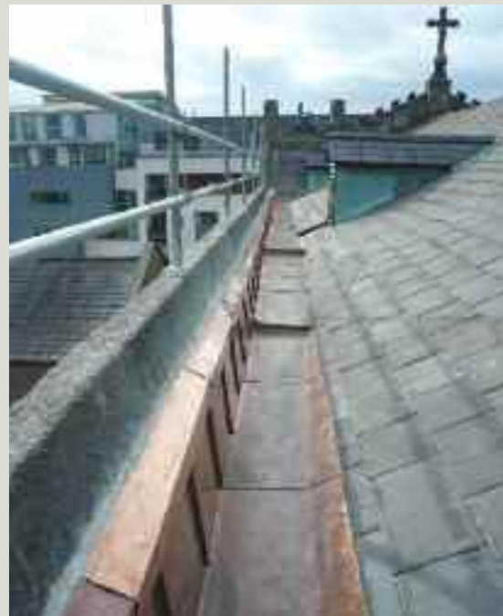
The failed copper guttering and parapet flashings on this church (left) were replaced with new copper guttering and flashing and the stone cleared of growth (right). The snow, or access, boards were not replaced as these can constitute a significant trip or fall hazard at roof level, particularly when they are in poor condition
