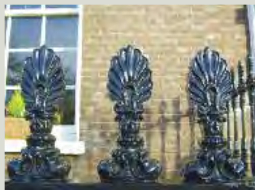
Mid nineteenth-century railings with wrought iron bars and rails, and decorative cast iron finials and husks
