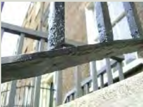
Where new rails are installed, traditional detailing should be matched where possible, such as piercing bars through the rail
