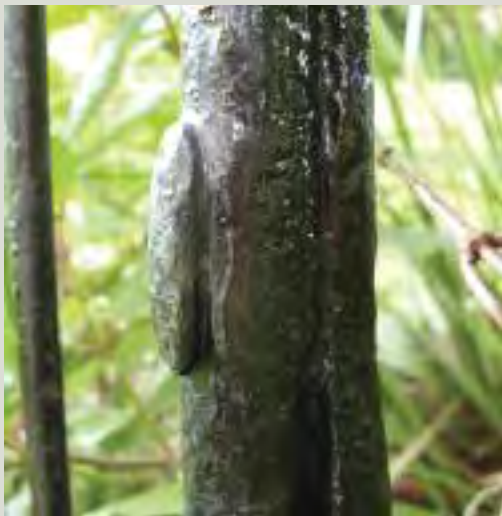
Original wrought iron backstay fixed in place by means of a bradded (riveted) pin
