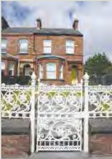
Cast iron railings and gate, Limerick
