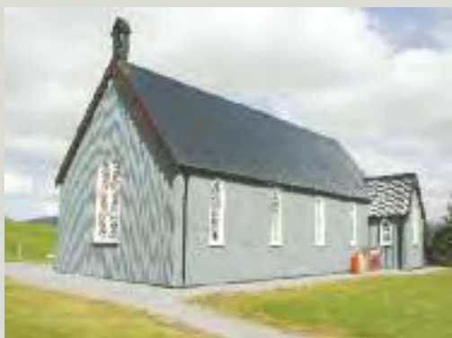
Lurganboy Church of Ireland church, County Leitrim. A fine example of a corrugated-iron clad 'tin church' built in 1862
