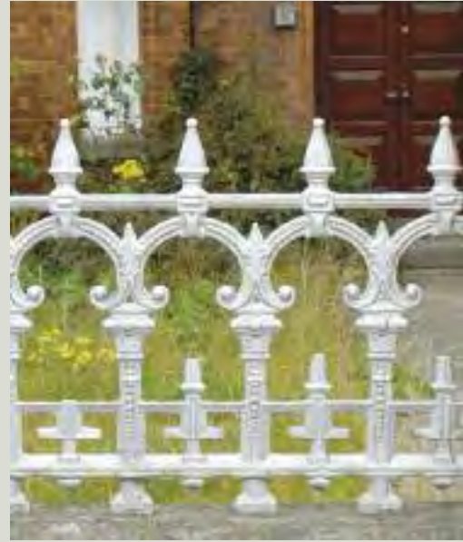
This design is typical of cast iron panels cast in repeating, identical sections. Patterns for railings such as these had to be designed so that there were no undercuts – it had to be possible to pull the pattern out of the sand mould without pulling away any of the sand (which would get trapped behind undercuts) in the process. Some panels have a taper from one side to the other which aided the removal of the pattern from the sand mould
