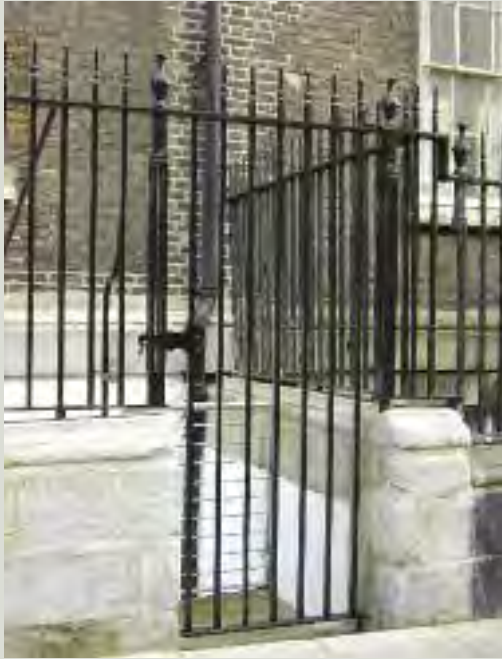
This replacement gate has been inserted sensitively and has been designed to tie in with the proportions and design of the original railings
