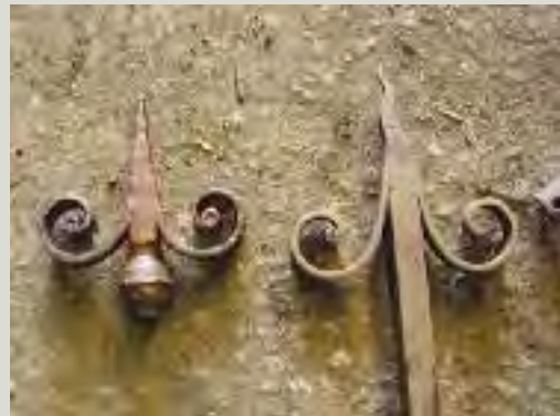
While modern welding techniques are not ideally suited to traditional ironwork, a skilled craftsman may be able to apply modern welding to repairs to a level that is visually acceptable. The finial on the left has been forge welded and hammered down to a point, while the finial on the right has been electric arc welded and then hammered into a point in the traditional way
