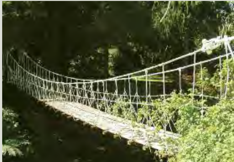
An early and unusual multiple-wire cable suspension bridge (1826) in the grounds of Birr Castle, County Offaly
