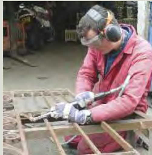
A needle gun can be effective at removing corrosion material, but can be damaging to the surface of ironwork if applied with too much pressure (Image courtesy of Historic Scotland)
