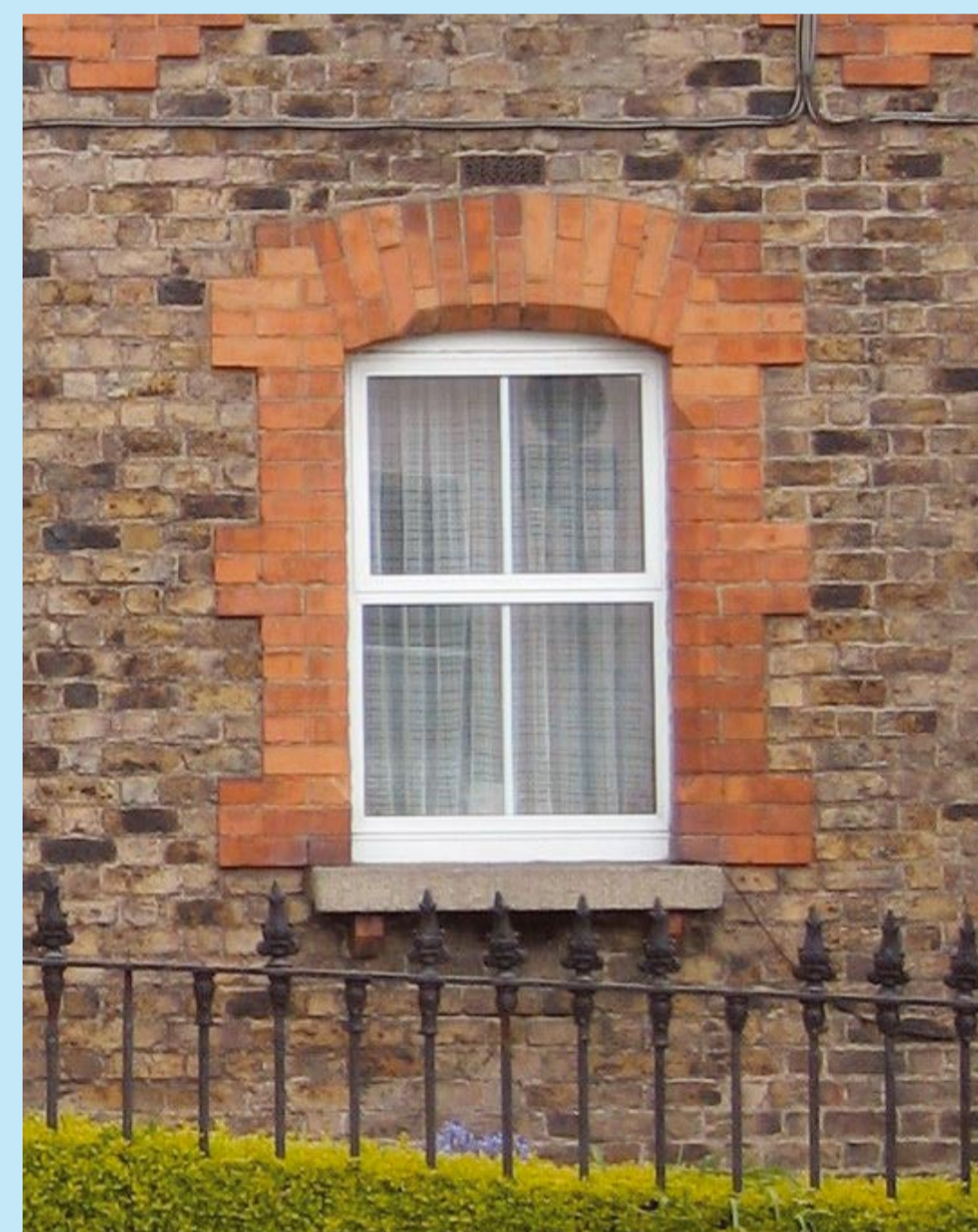
ABOVE: Above: Loss of original sash window
