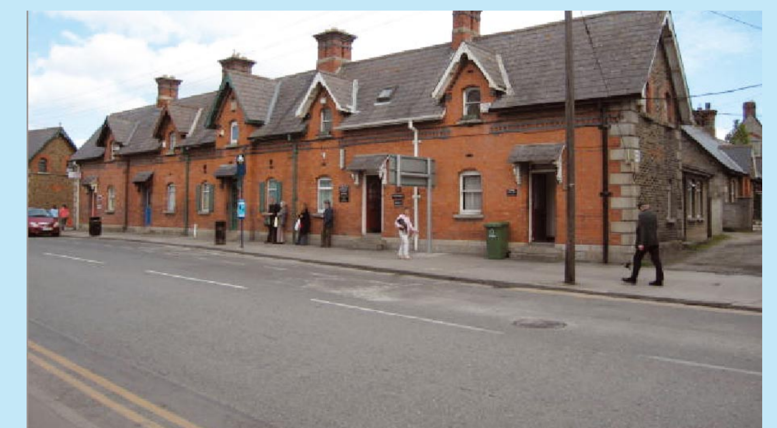
ABOVE: A view of Clarinda Park House from the west. This large five-bay two-storey over basement this is a landmark building in the park.
