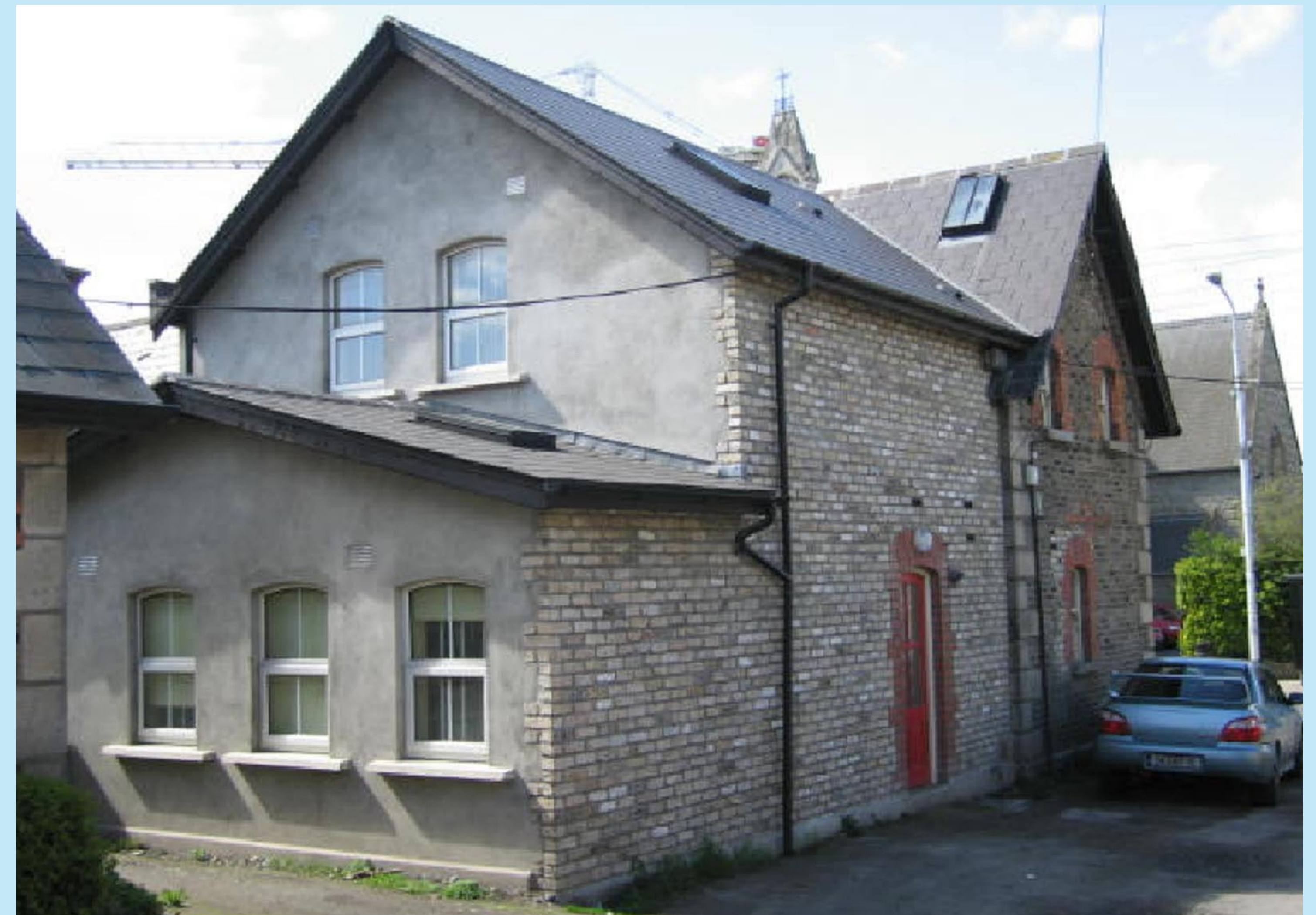
ABOVE: A view of Clarinda Park House from the west. This large five-bay two-storey over basement this is a landmark building in the park.
