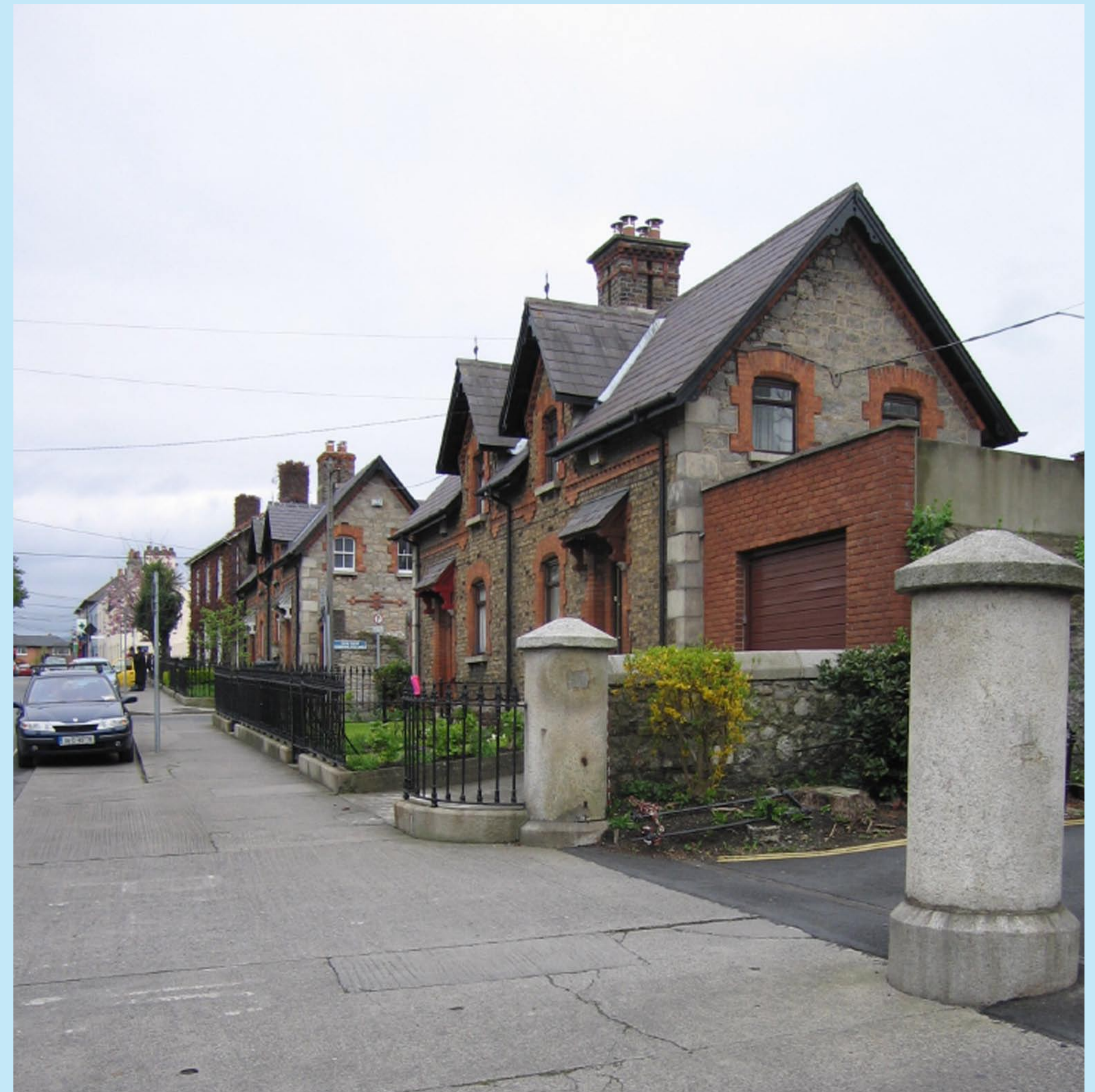
ABOVE: View of the Pembroke Cottages, Booterstown Avenue
