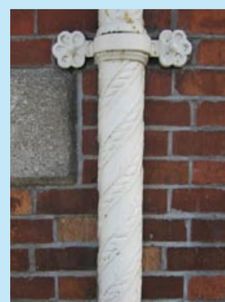
ABOVE: Spiral fluted cast-iron downpipe
