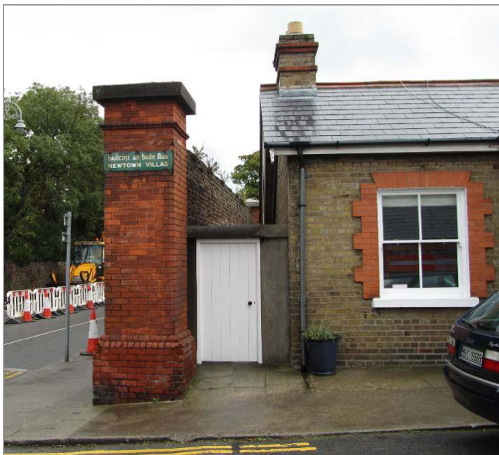
Lane access gate (beside No. 1) with a view of the brick inner lining of the former garden wall.
