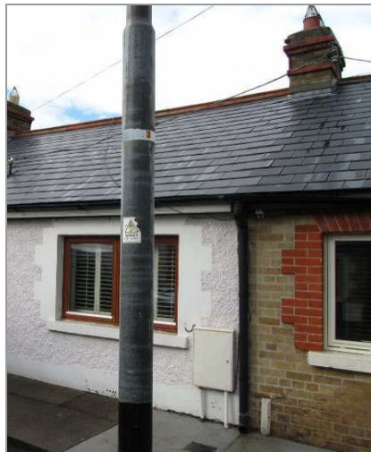
L: obtrusive large surface mounted meter box
