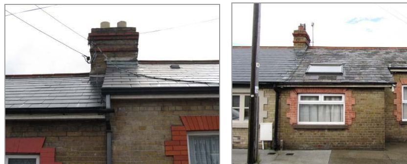
left: electricity cables trailing over roofs from chimneys
