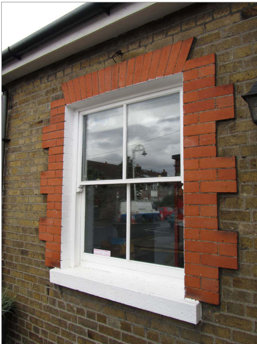
Brick reveals to windows arranged as quoins with flat arch above
