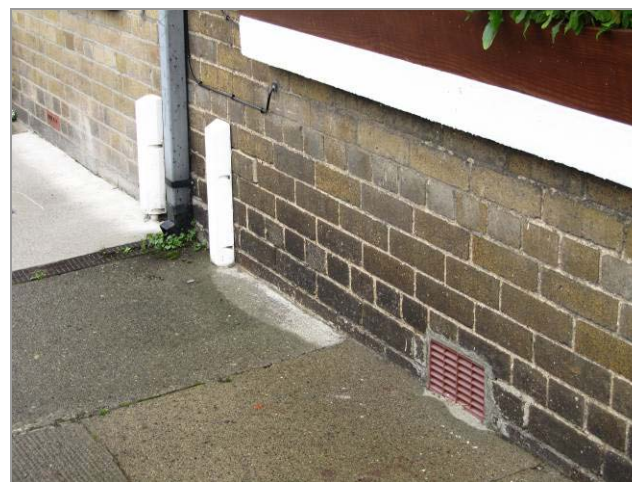
Replacement of ventilation bricks with plastic grill
