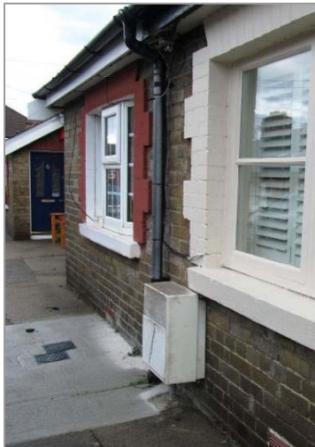
L: obtrusive large surface mounted meter box
