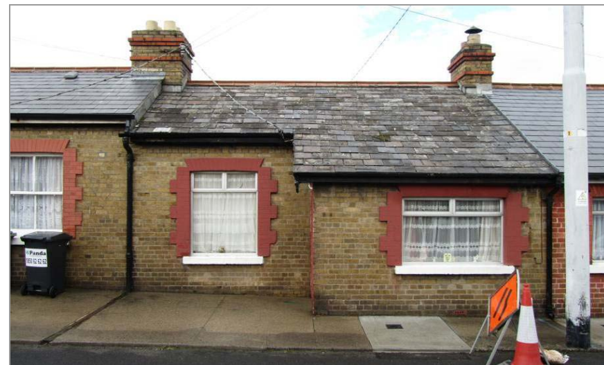
Roof with original natural slates
