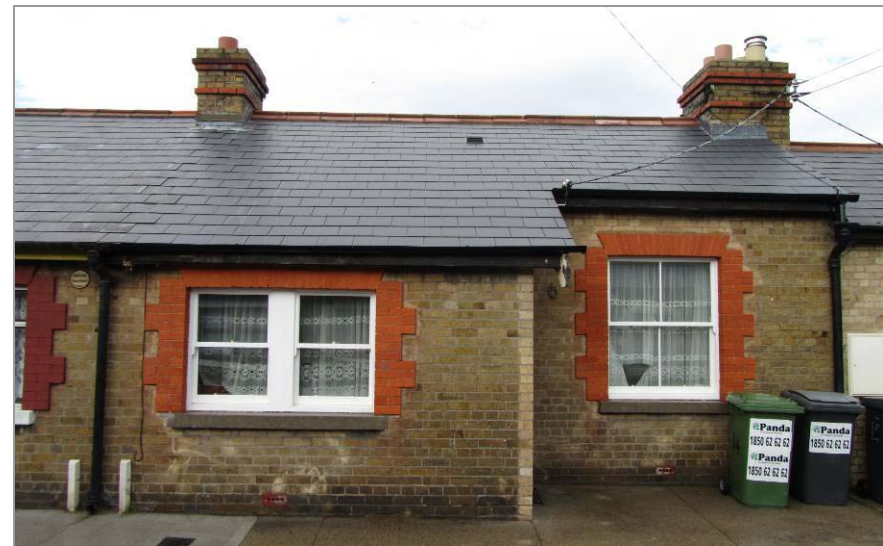
Original sash windows
