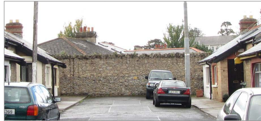
Stone wall of former garden at the south end of Newtown Villas
