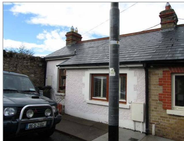
Render applied to a brick elevation
