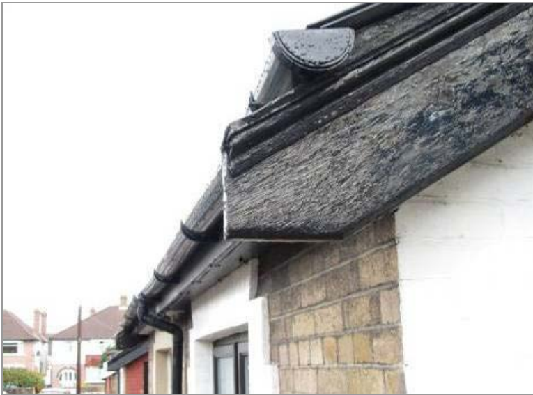
Barge board detail with moulded profiles
