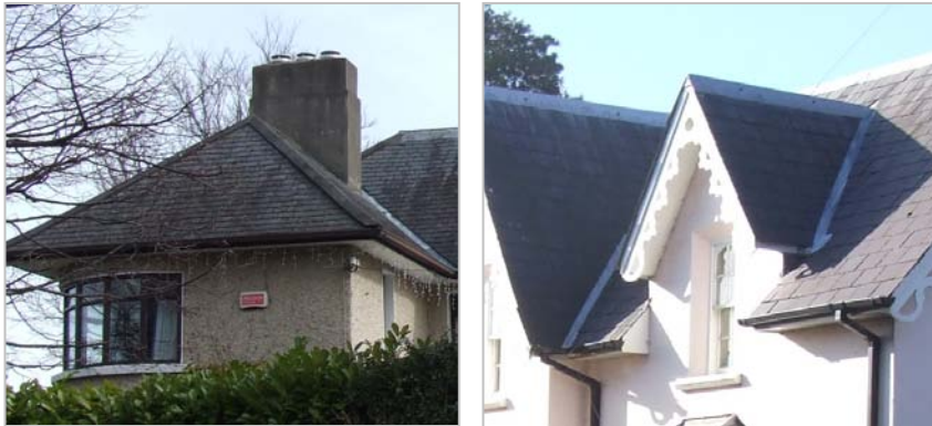
A natural Slate finish covers the majority of the roofs
