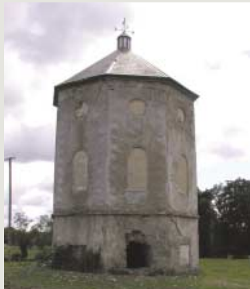
The original roof of this eighteenth-century dovecote was lost; however sufficient evidence survived to design a new roof which complements the structure
