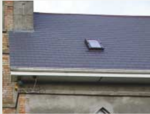
Inappropriate alterations to roof shapes and details detract from the character of a structure; in this case the new roof has overhanging eaves with uPVC fascias, soffits and rainwater goods - an incorrect design using inappropriate materials on this former Board of First Fruits church
