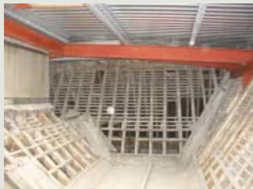
Old roof timbers should not be routinely stripped out as this can lead to a loss of character and the destruction of important historic elements. In this case, a roof structure, dated to the 1580s using dendrochronology, remains intact and, although no longer capable of taking the weight of cladding, is preserved beneath a new metal structure
