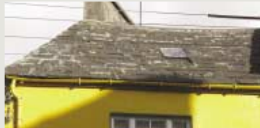
Moher 'slates', a regional type of roof cladding once common in Co. Clare, are in fact thin slabs of limestone dressed as slates. Stone 'slates' are rare survivors and, wherever possible, should be maintained in place with minimum intervention
