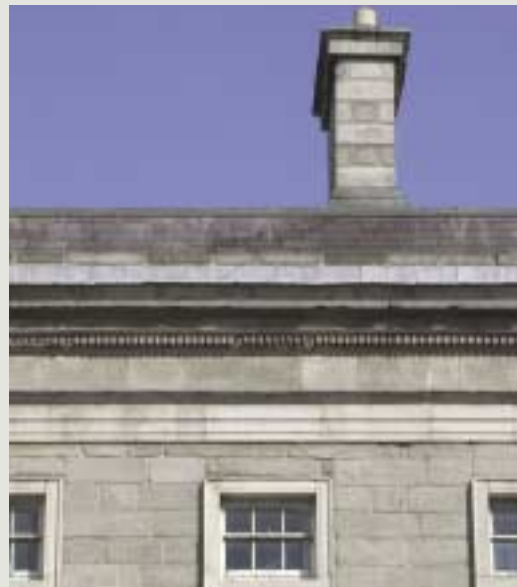
The eaves of a building can be vulnerable to weather-related problems, typically parapet walls become saturated as they are exposed on both sides to rain. Problems will also arise where the blockage of the gutter concealed behind a parapet may not be readily noticed. However, where they exist, parapet walls are usually an important architectural feature of the building
