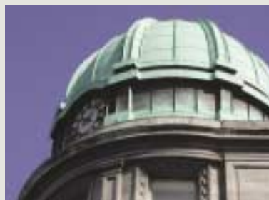
The visual impact of domes, lanterns, steeples and other prominent architectural features can extend well beyond their immediate setting and their removal may affect a wide area even where they are unused or unnecessary to the current use of the building
