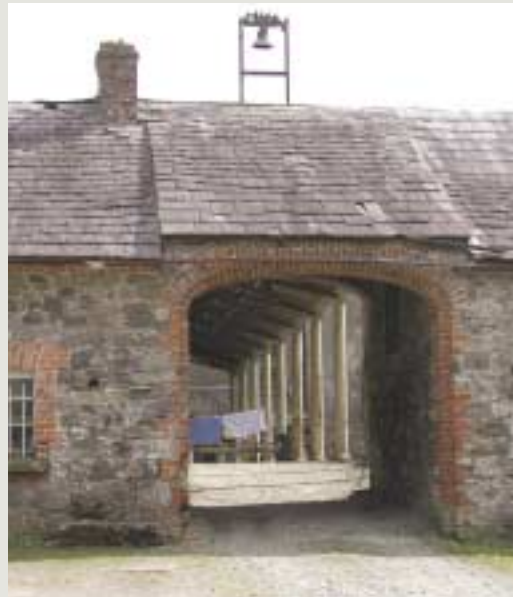
Undulations and previous repairs of good quality may all contribute to the character of a roof. Any necessary works should leave intact original detailing such as this raised archway roof, as it provides definition to the entrance bay
