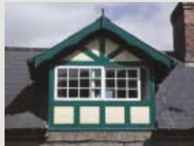
Original dormer windows were usually designed as part of the architectural vocabulary of a structure and may contain a wealth of detail such as finials, ridge tiles, bargeboards and slate-hung or glazed cheeks
