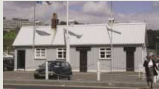
Corrugated iron sheeting may degrade through cracking or rusting (caused for example by sea spray in maritime areas) to a point where replacement is necessary. This recently-reclad harbour-master's office has replaced the original, but rusting, corrugated iron with a modern profiled metal sheeting
