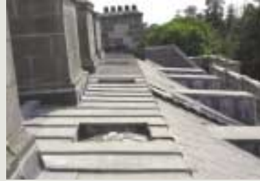
Lead or copper sheeting were traditionally used on flat roofs or as a cladding to domes or cupolas. Lead, if properly specified and laid, can last several centuries in situ. Lead flashings can sometimes be cut with decorative finishes. Leadwork may have dates or inscriptions scratched on as graffiti, which is now of historical interest
