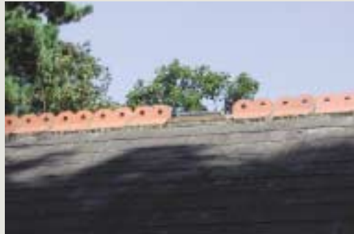
Where it is proposed to ventilate roof spaces, important architectural details should be retained intact; in this example a pierced ceramic tile has been replaced by a new vent tile which disrupts the line of the ridge comb and damages its visual integrity
