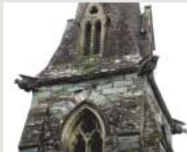
Masonry details associated with roofs may be functional or not. Whether they are plain or decoratively detailed, they add character to a roof and, even if now redundant, should be retained
