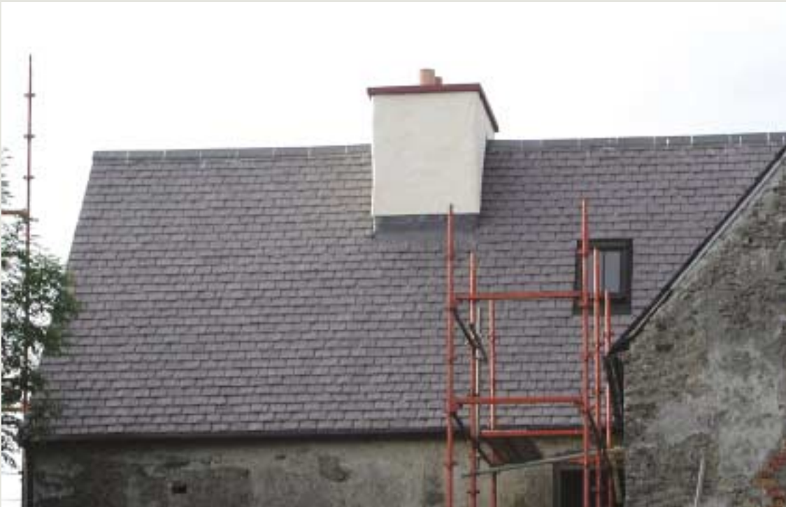
Valentia slate, famed for its qualities during the nineteenth century and again being quarried on a commercial basis, is here used on a conservation project. The use of regional slate types can be an important aspect of local distinctiveness and research indicates that slate native to a region generally performs best in the climatic conditions of that area. When undertaking restoration works to important roofs, the feasibility of reopening a local quarry to supply new slate should be investigated
