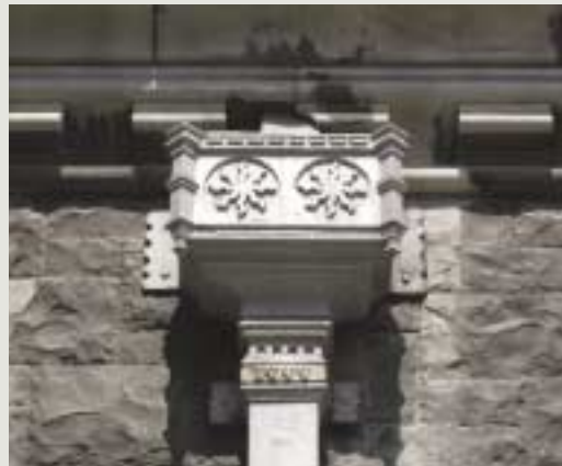
Good conservation practice encourages the honesty of repairs and alterations which may be discernible to the expert eye but not visually obtrusive. This new hopper head was designed to match the style of the structure but is recognisable, on close inspection, as a new element from its 1999 date
