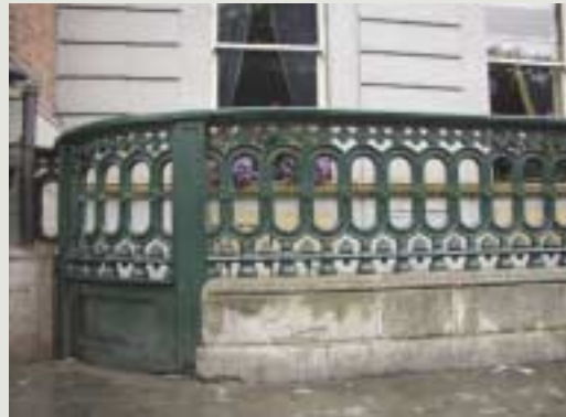
The careful repair of a damaged feature such as a cast iron balustrade contributes much to preserving the character of a structure (shown here before and after repair). Where elements are not capable of repair, the new work should accurately reproduce the detail of the original. Entire sections should not be replaced if only a part is damaged
