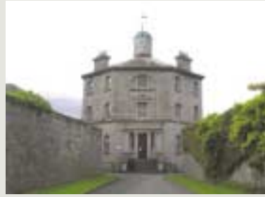
Buildings should be kept in active use, preferably the original use. Where this is not possible, permitted changes of use should aim to minimise the impact on the character of the structure, as with this former gaol observation tower, which is now in education-related office use
