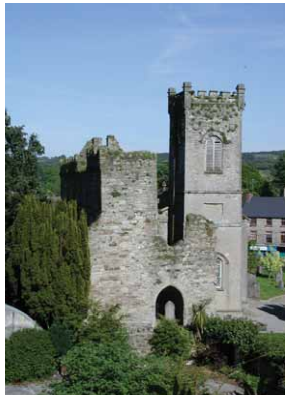
Some redundant churches are also recorded monuments, or are within the area of constraint around the monument: they may be on the site of, beside or in the midst of ecclesiastical remains. This former Board of First Fruits church was built partly within the walls of a mediaeval church that is now a National Monument in state guardianship
