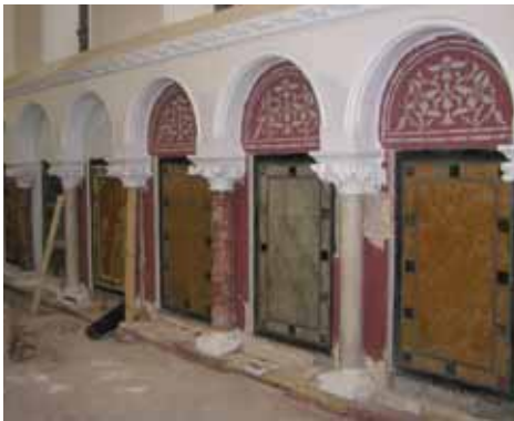
In this example, the original decorative paint scheme is being recreated based on detailed evidence
