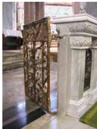
Internal fixtures such as box pews, confessional boxes and altar rails can be significant elements of the character of the place of public worship
