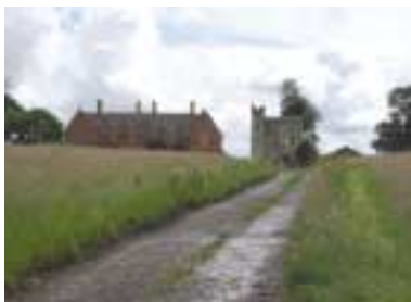
There may be other structures nearby which have an association with the structure that is the subject of the inspection and will contribute to a fuller understanding of the site, such as earlier houses, castles or industrial remains
