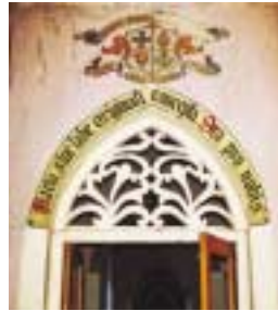
In these examples, interior features of importance have been damaged and any proposed repair will require to be carried out to a high standard in order for the work to be considered exempted development
