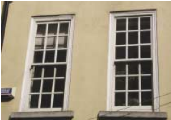
These replacement windows, although in many respects well detailed, have horns on the sashes, which is incorrect for the period of the building
