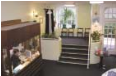
The careful removal of later alterations of little interest, such as this half floor and steps, may be exempted by a declaration
