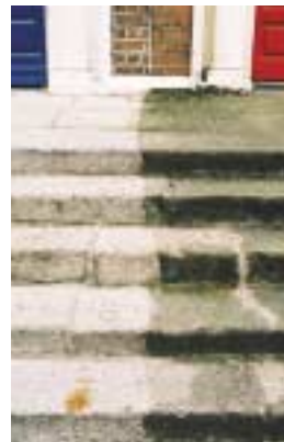
Uncoordinated programmes of stone cleaning can create aesthetic problems in terraces of similar buildings
