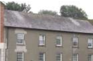
The removal of chimney stacks can damage the appearance of an entire building
