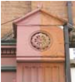
The application, and subsequent removal, of paint from terracotta (and soft stones such as sandstone) can cause damage to the material and jeopardise its future conservation
