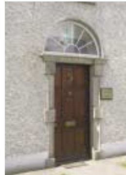
The replacement of original features, in this case the fanlight and door, with substitutes made from inappropriate materials should not be considered exempt
