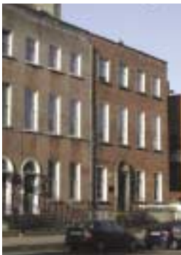
The rendering of the terraced building on the left has altered the character, not only of the individual building, but of a terrace of protected structures
