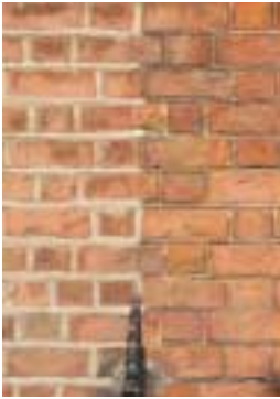
Repointing which uses methods and materials other than the originals may alter the character of the building as has happened with the example on the left of this photograph
