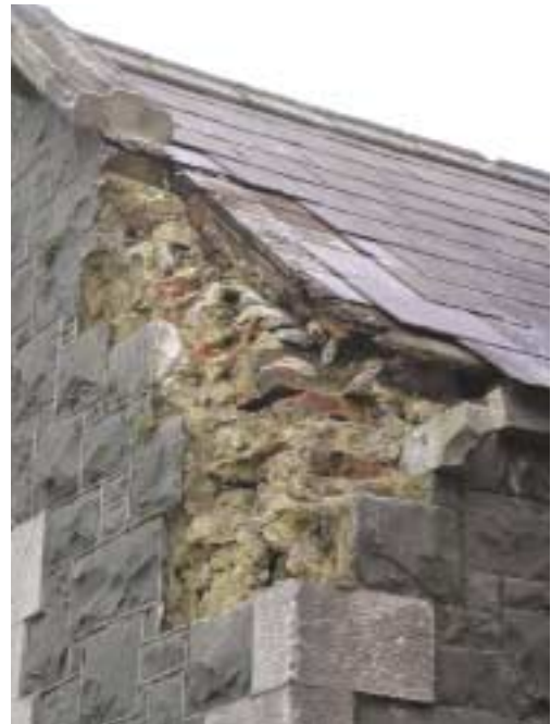
Urgent works may be needed to secure the fabric of a building following damage
