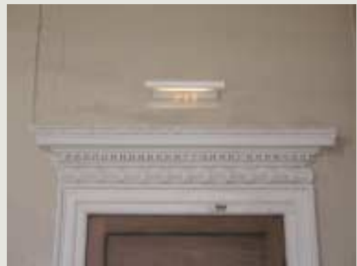
The use of standard signage may not be appropriate in high-quality interiors. Alternative designs are available which minimise the visual impact while fulfilling fire-safety obligations
