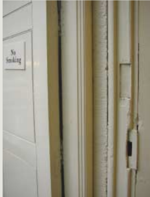
The reversal of a door to allow it to open in a different direction may require obtrusive alterations to a historic doorcase and may make the original hinges and locks redundant
