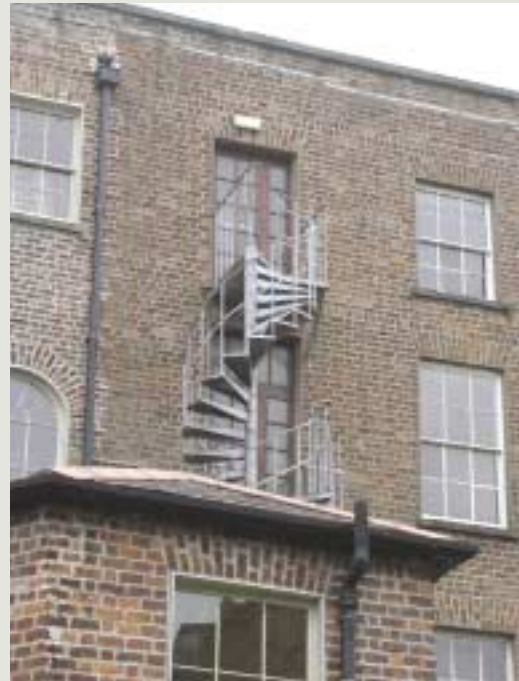
Proposals that require the conversion of original window openings into doors to facilitate escape will require very careful consideration and should avoid impacting on surviving early or original windows and on important elevations. There may also be a potential impact on nearby windows which may require re-glazing with fire resistant glass
