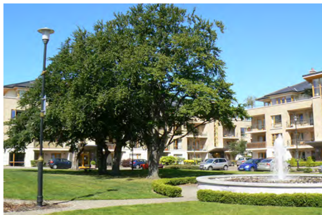
Photo : 11 Trees incorporated into Trimbleston Development, Goatstown
