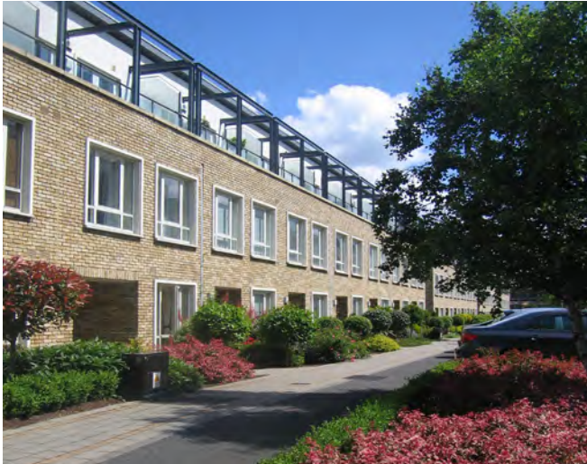
Photo 16: Example of Three-Storey Residential Development
