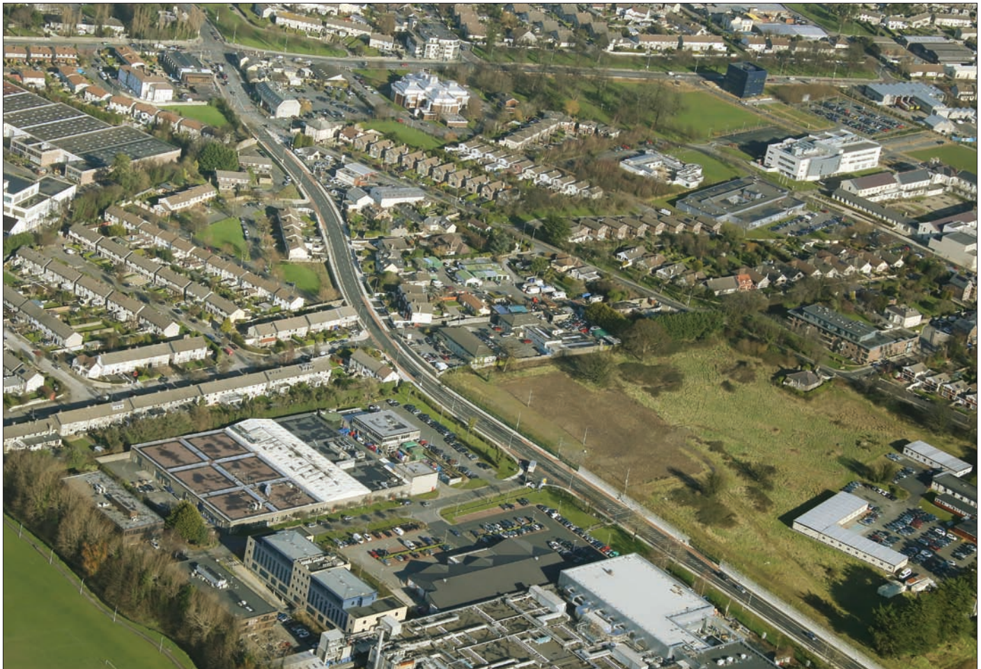
Aerial View of Pottery Road Improvement Scheme
