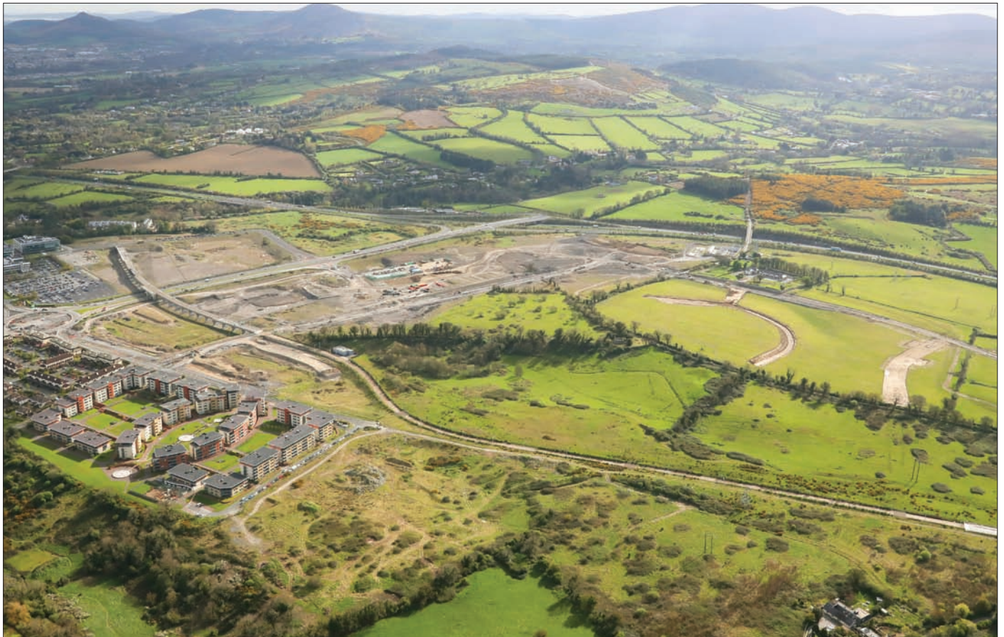
Aerial View of Cherrywood SDZ
