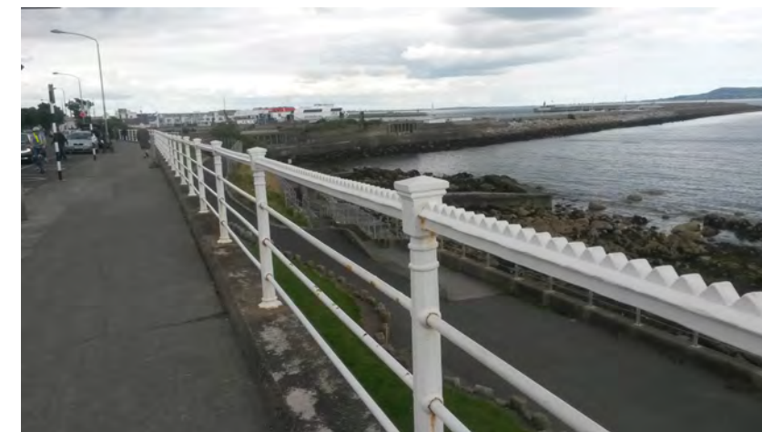
Photo 25: Railings along Queen's Road, Dún Laoghaire.
