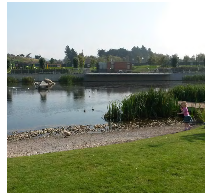
Photo 37: Attenuation Feature at Honeypark, Glenageary.
