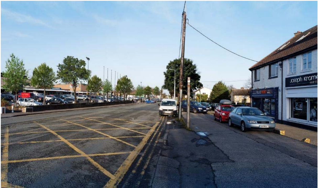
Figure 10.10: Old Dublin Road Currently (South section)
